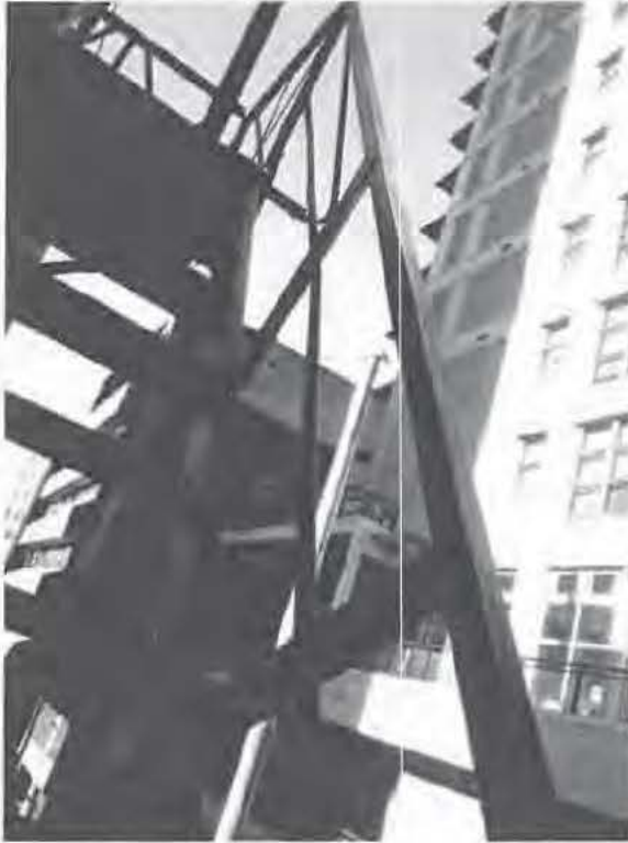
Figure 5, Broken connection between the east guard and fire escape stair.
