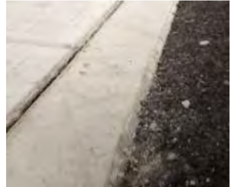
Figure 4 - Damage to the Lower Edge of Curb B from the Asphalt Roller
