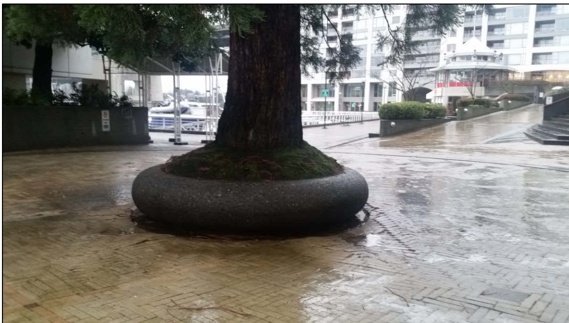
The base of the tree showing the limited space within the planter and the root damage to the paved areas.
