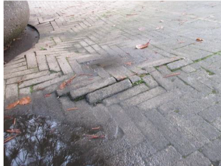
Photo 3: Uneven pavers around planter.
