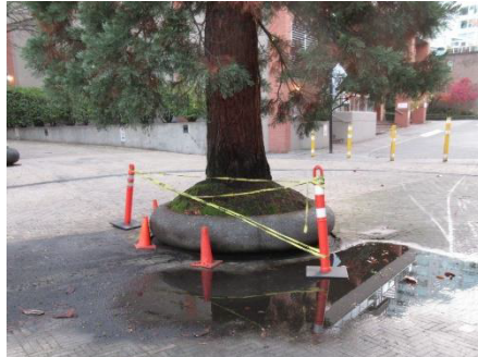
Photo 2: Ponding water around planter.
