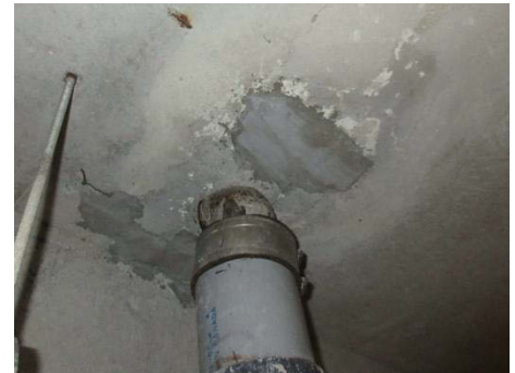
Photo 4: Efflorescence and previous concrete repairs below the tree.
