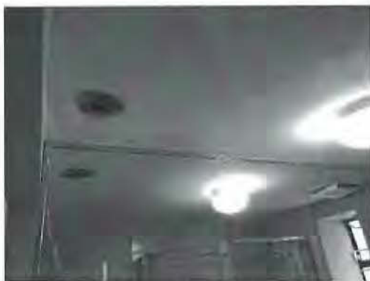
Lower Washroom - Mould on Drywall Ceiling
