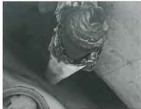
Mechanical/Boiler Room - Asbestos Pipe Insulation
