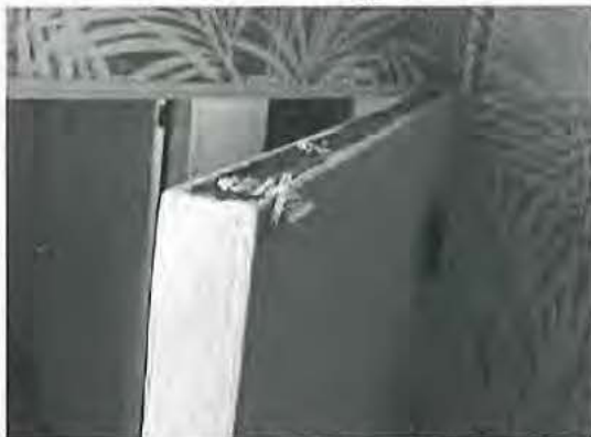
Upper-Level Main Washroom – Wood Door – Lead Paint
