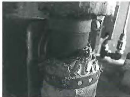
Mechanical/Boiler Room - Asbestos Pipe Insulation
