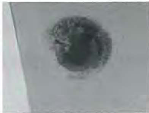
Lower Washroom - Mould on Drywall Ceiling
