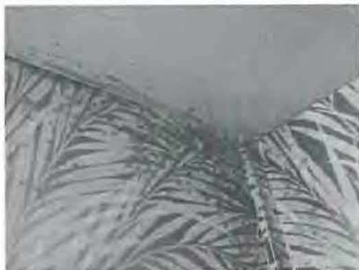
Upper Washroom - Mould on Drywall Ceiling and Wallpaper
