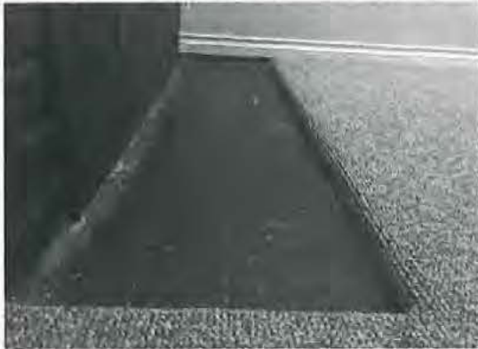
Lower Level West Bedroom – Fireplace Hearth – Lead Paint
