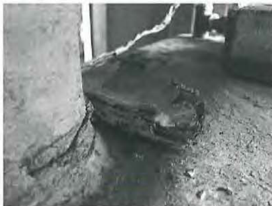
Mechanical/Boiler Room - Asbestos Pipe Insulation Debris
