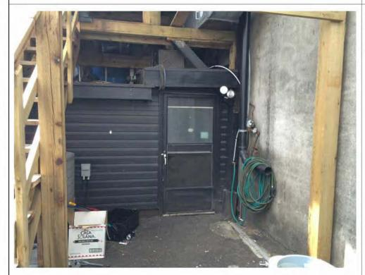
Exterior storage & cooler behind, deck/stair and noncomplying kitchen exhaust duct wwop.
