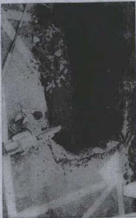
② VIEW OF TOP OF EXPOSED TANK; BADLY DEFORMED. CONTAMINATED SOIL SUSPECTED.
