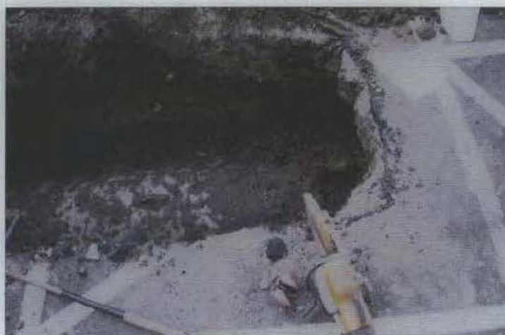
② VIEW OF TOP OF EXPOSED TANK; BADLY PERFORATED. CONTAMINATED SOIL SUSPECTED.
