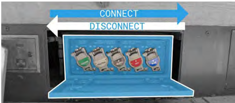
3. Working in sequence LEFT to RIGHT , lift each coloured flap in turn and install the matching coloured cable before moving to the next cable until all 5 are connected:
