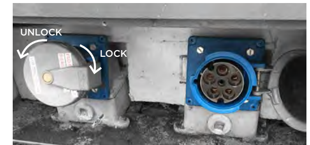
3. Open lid and attach cable to receptacle. To unlock lid: turn left / To lock: turn right. Consult Security for proper cables.
