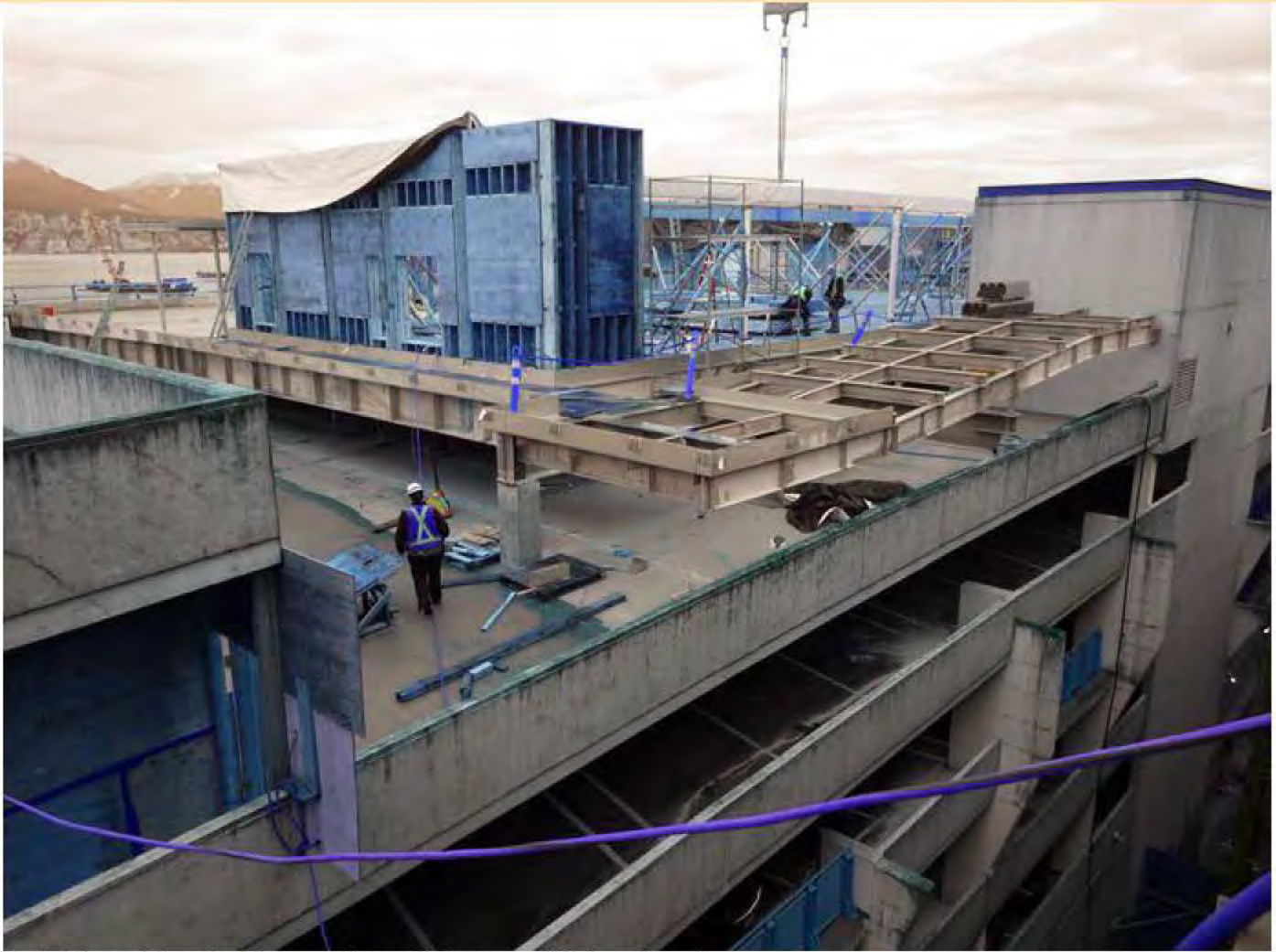
Prefabricated Passive House wall panels/"cassettes" being placed
