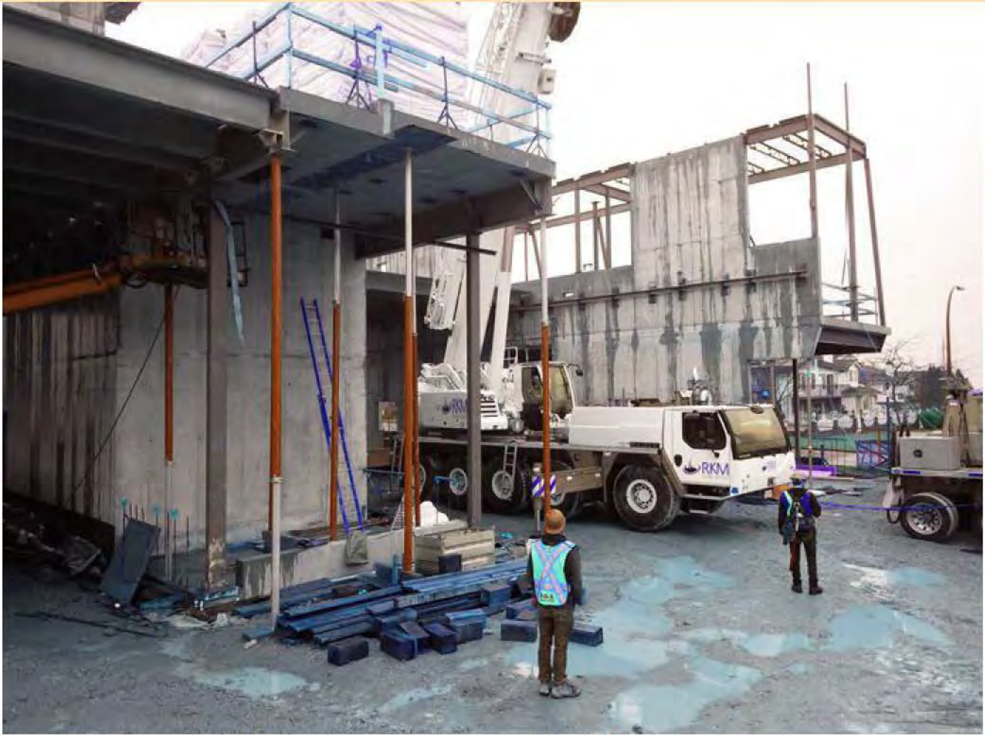
Crane truck in Apparatus Bay location placing precast concrete double "T" beams
