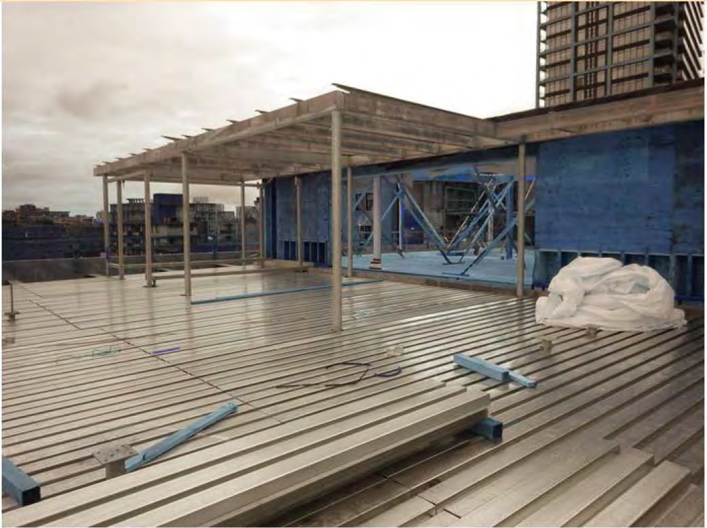
Framing for covered and uncovered exterior play area
