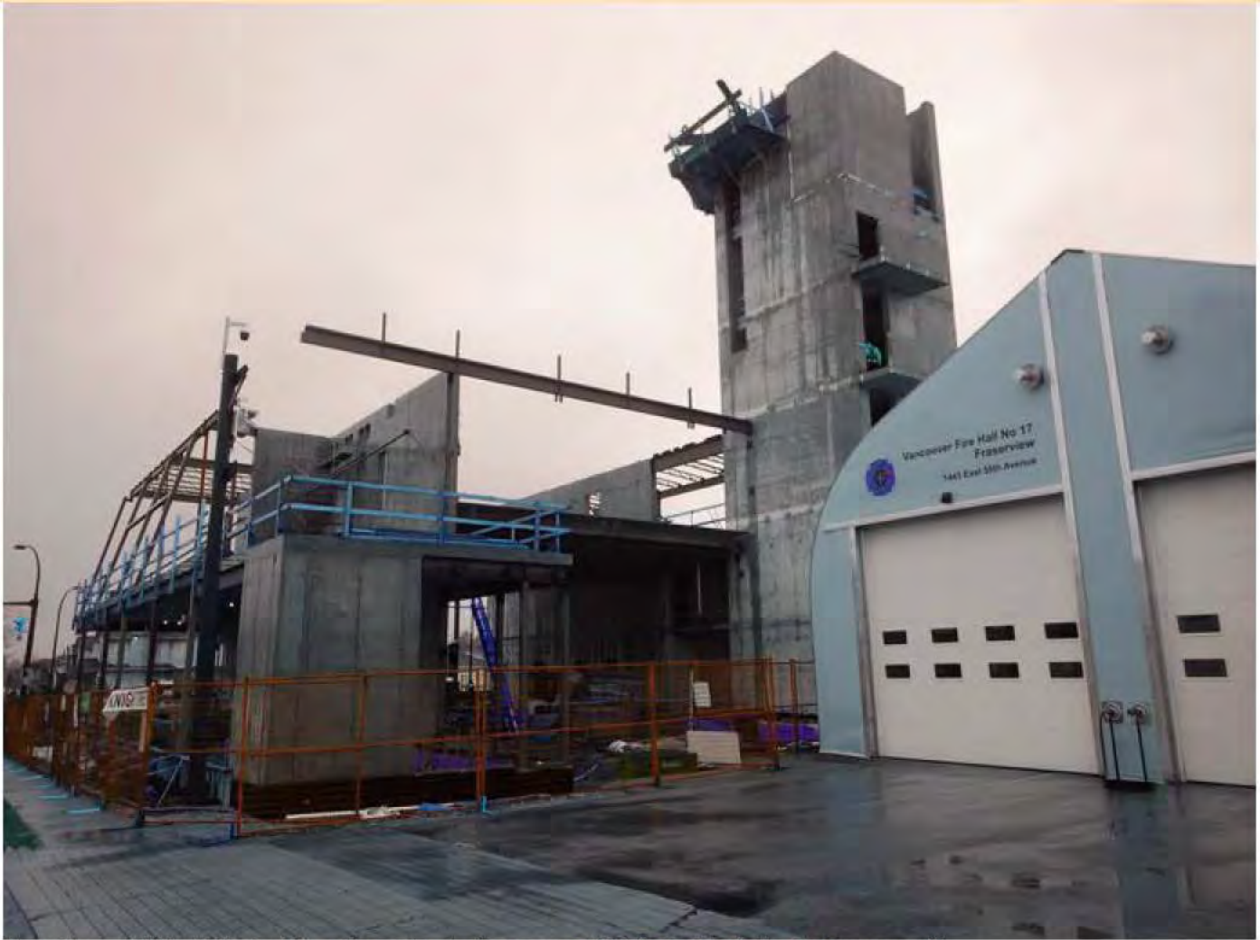
Hose tower full height; steel framing going in (temporary FH 17 truck shelter in foreground)
