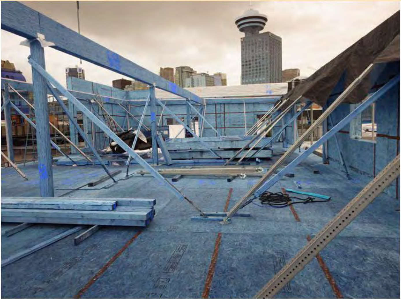
Prefabricated Passive House panels/"cassettes" and composite wood posts and beams
