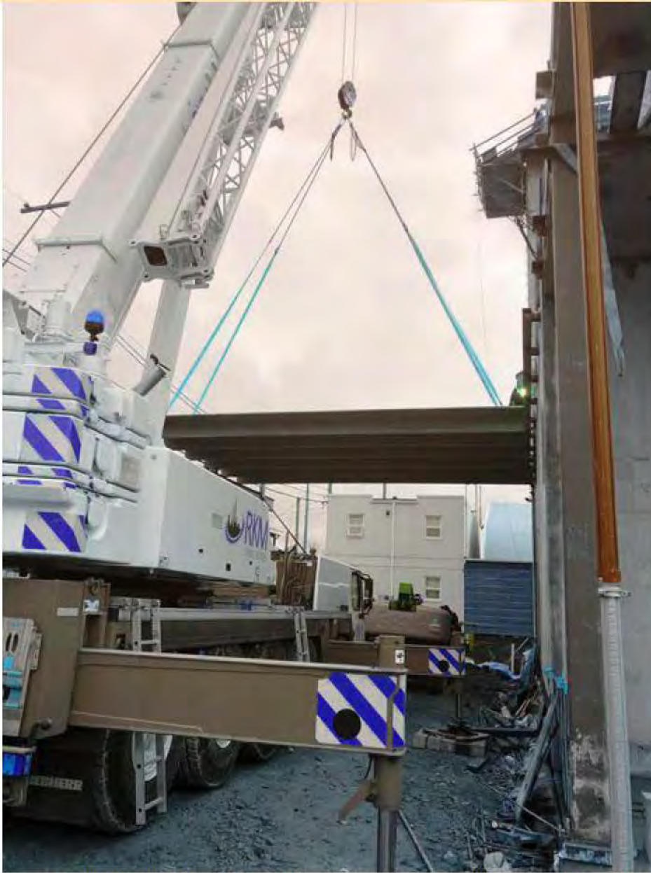
Concrete double "T" beams being placed above Apparatus Bay (temporary FH 17 quarters in background)
