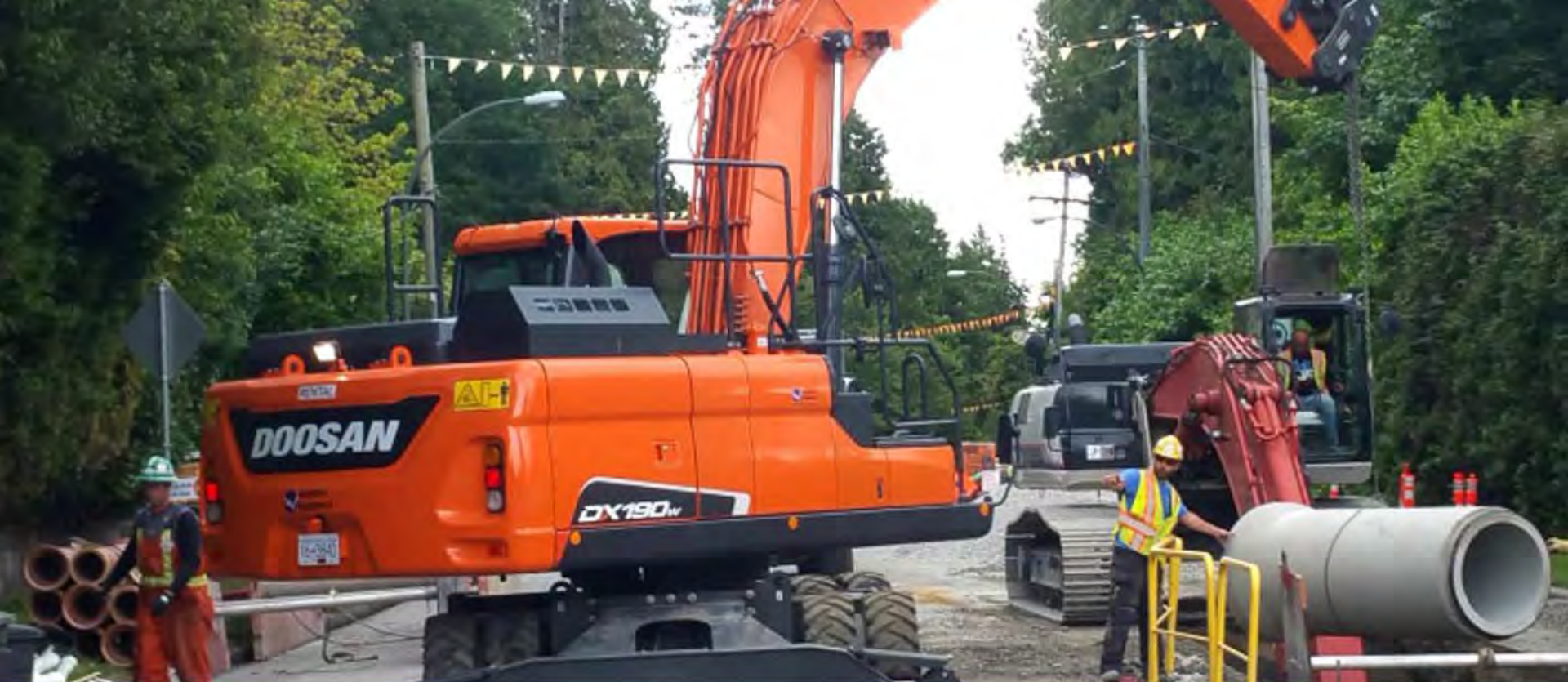
Above: Sewer Operation crews install a separated sewer on SW Marine Drive.
