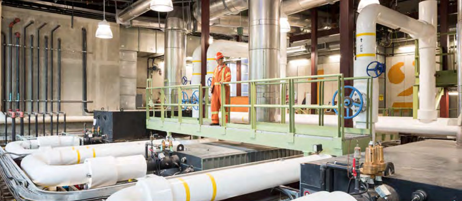
Above: Staff of the Southeast False Creek Neighbourhood Energy Utility (NEU) look over the two massive heat-transfer units. The NEU was the fourth sewer heat recovery system in the world.
