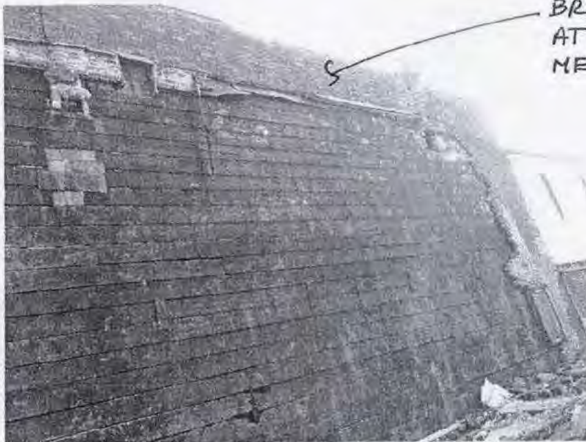
Figure 11: Brick Veneer Intact on East Elevation of 439 Powell Street, Vancouver
