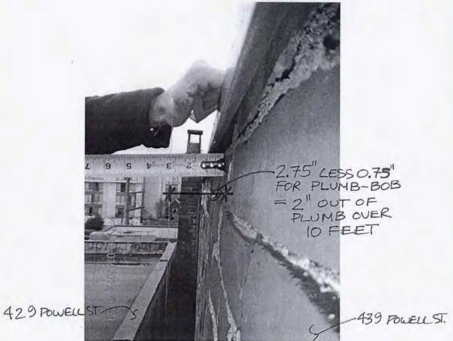
Figure 13: Brick Veneer Out of Plumb on West Elevation of 439 Powell Street, Vancouver
