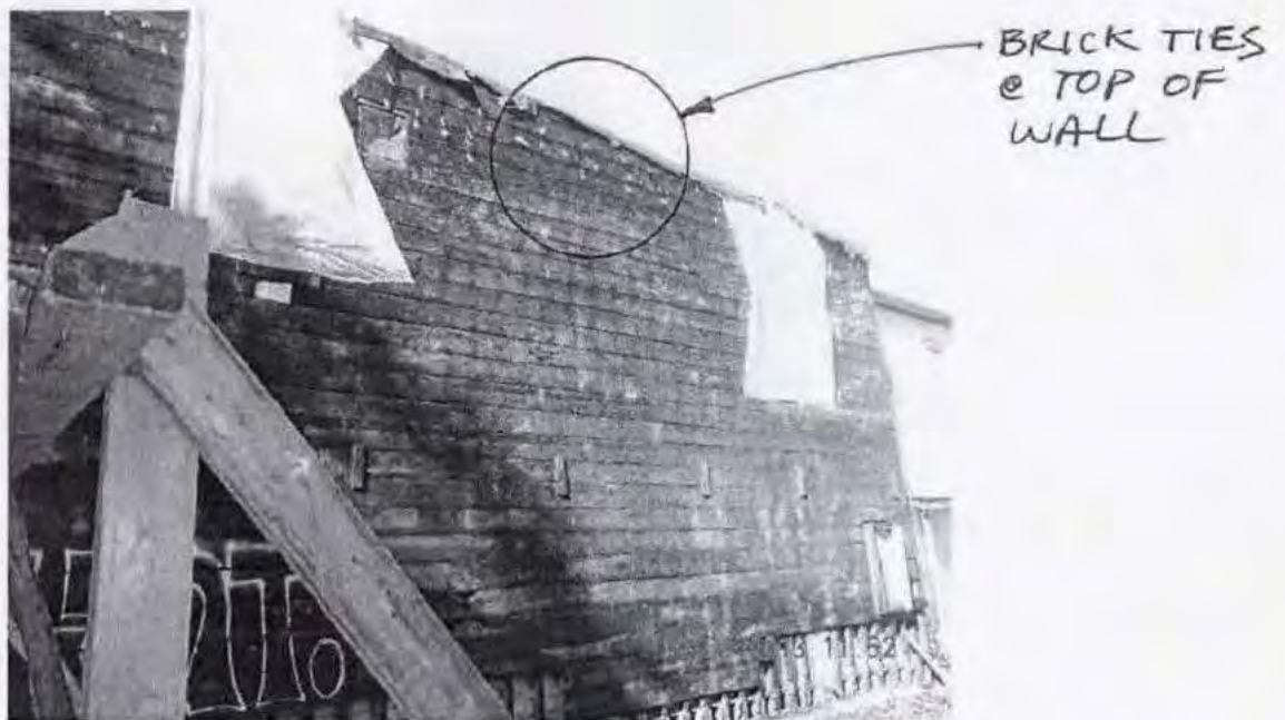
Figure 6: Brick Ties for Anchoring Brick Veneer to East Wall of 439 Powell Street, Vancouver
