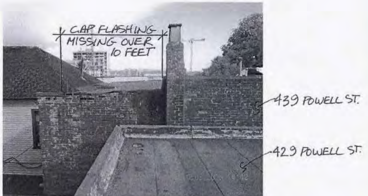
Figure 14: Cap Flashing Missing on West Elevation of 439 Powell Street, Vancouver
