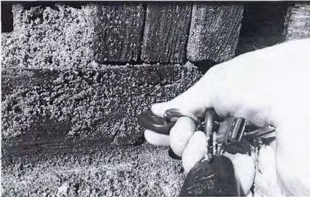
Figure 10: Key Fully Inserted into Wood Plate of East Wall of 439 Powell Street, Vancouver
