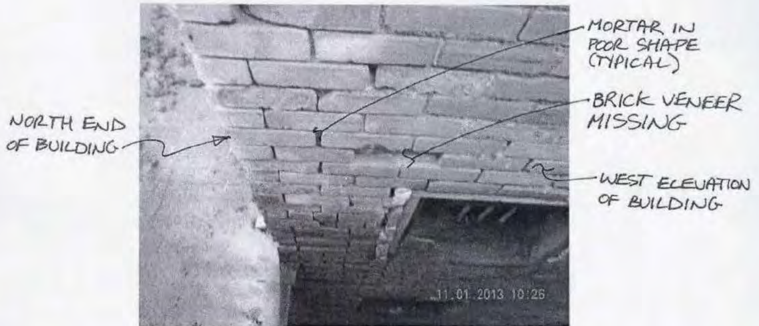
Figure 16: Mortar in Poor Shape at N-W Corner of 439 Powell Street, Vancouver
