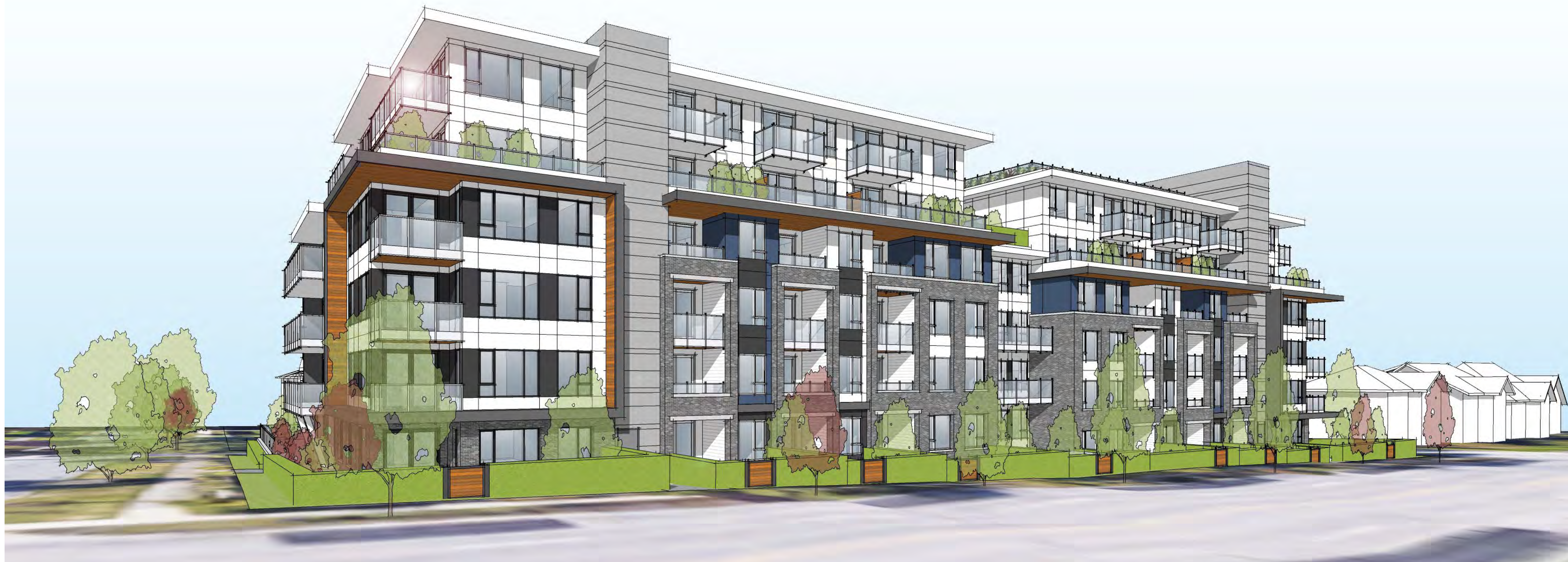
ARBUTUS STREET - SOUTH EAST CORNER
