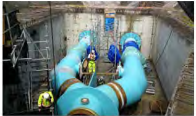
Pipe installation inside underground valve chamber
