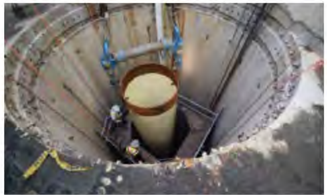
Water main installation through the shaft
