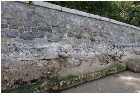
Stabilizing Undermined Foundations
