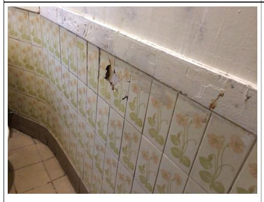
5<sup>th</sup> floor - west side w/c wall tiles damaged.
