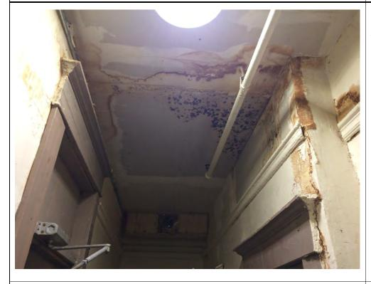
Example of water damage. Repairs made to wall finishes but water leaks still persist.
