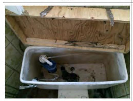
6th floor East side toilet showing broken and missing internal parts. The tank will not fill.
