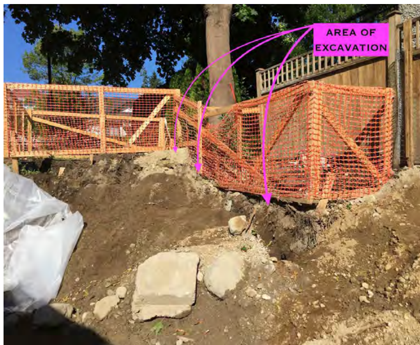
Tree #68 – site conditions – loose soil @ excavation wall
