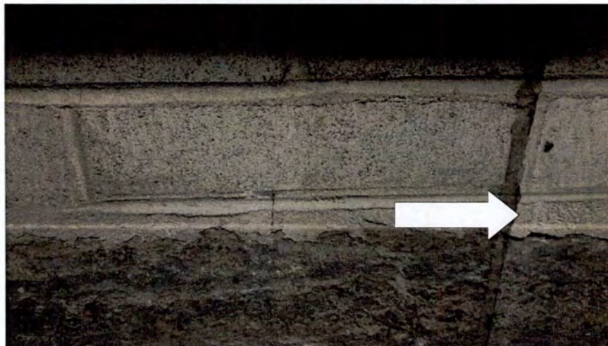
Residual Asbestos Containing Duct Mastic on Wall in Fan Room 024
