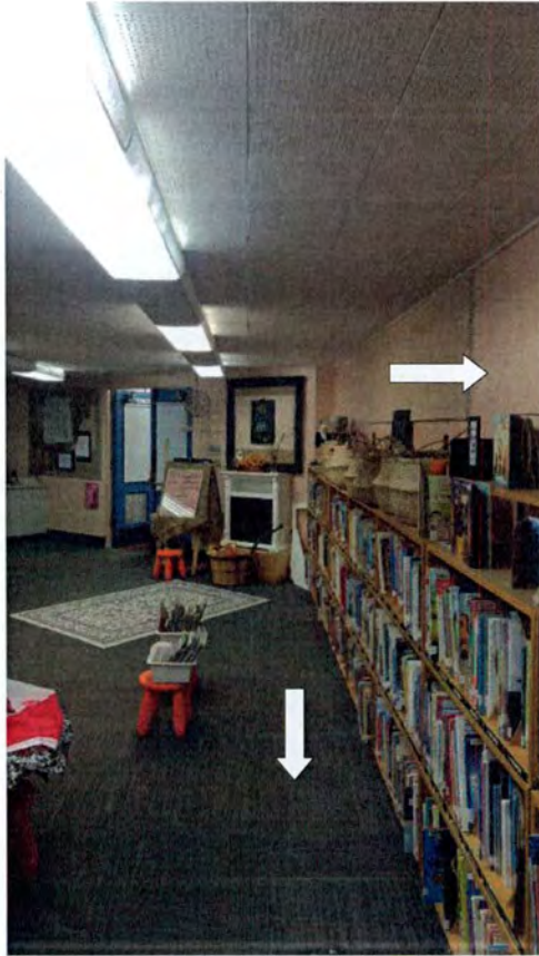
Asbestos Containing Drywall and Vinyl Floor Tiles (under carpet) in Library
