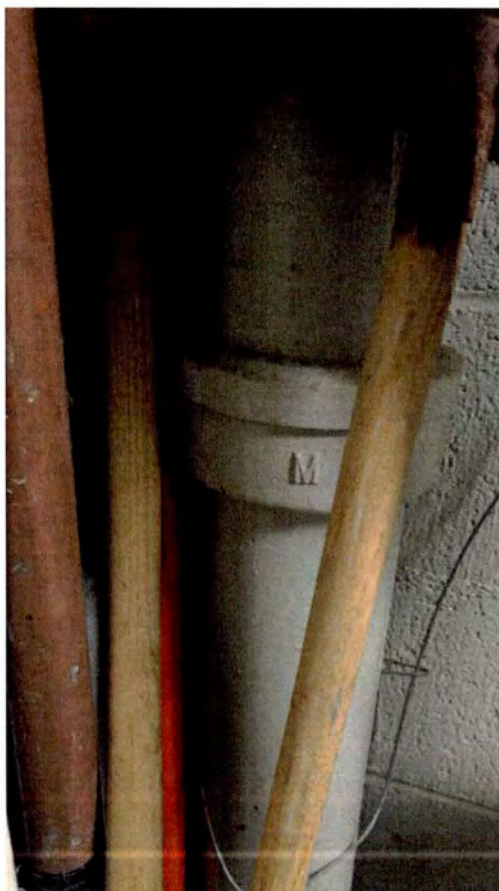
Assumed Asbestos Containing Bells & Spigots on Drain Lines
