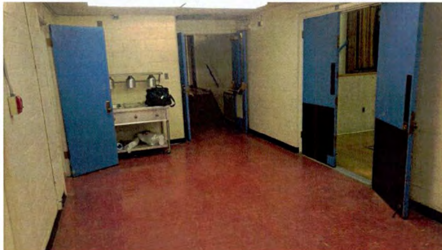
Corridor 023 – 9" Asbestos Red Vinyl Floor Tiles
