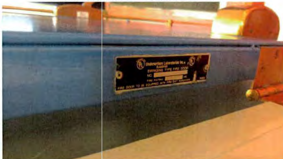
Assumed Asbestos Containing Fire Door Label
