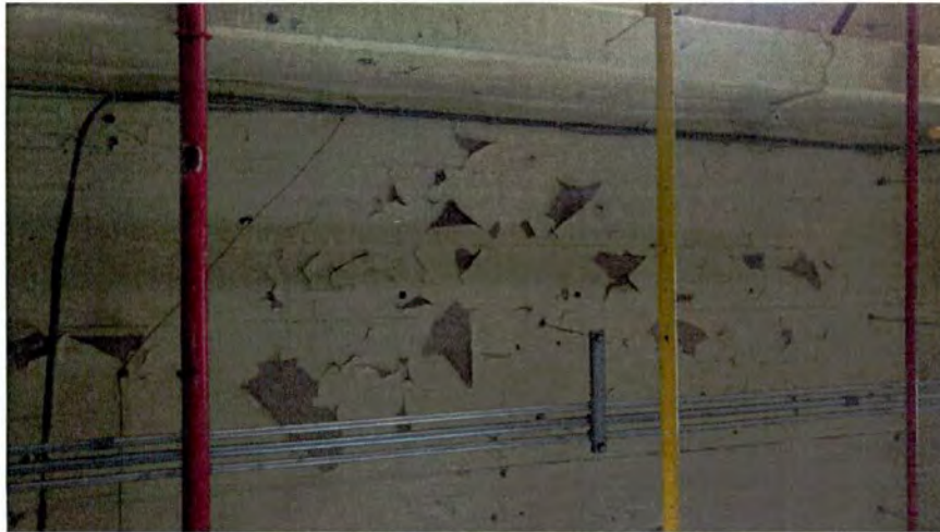
Peeling Lead Paint on Boiler Room Ceiling
