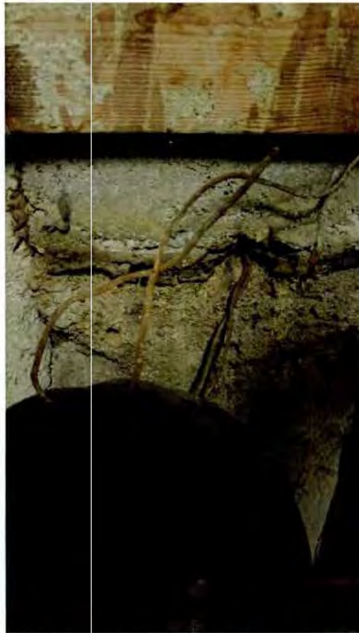
Asbestos Containing Wall Fill Material in Fan Room 024
