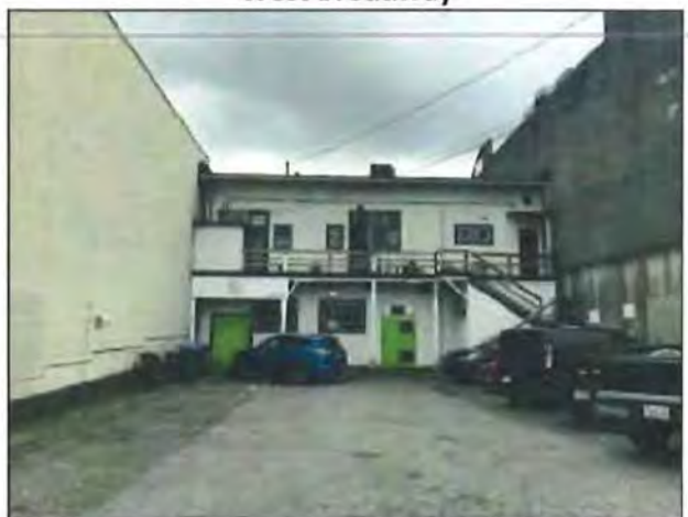
Rear Parking Area of Subject Site at 1441 West Broadway
