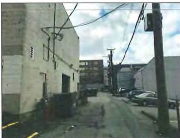
Western View of Rear Lane, 1431 West Broadway to the Left
