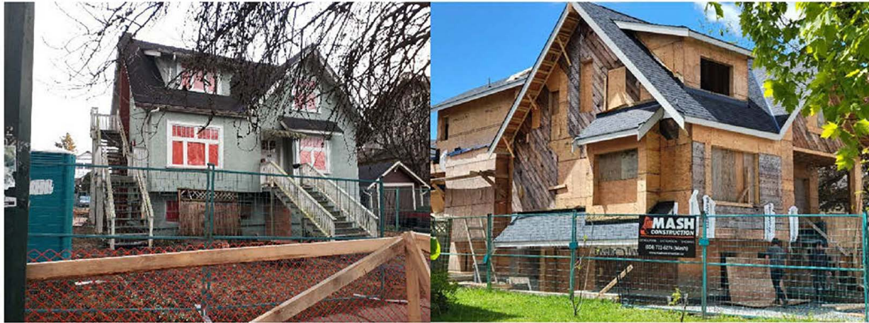
Figure 1: Character house retention and conversion project under construction
