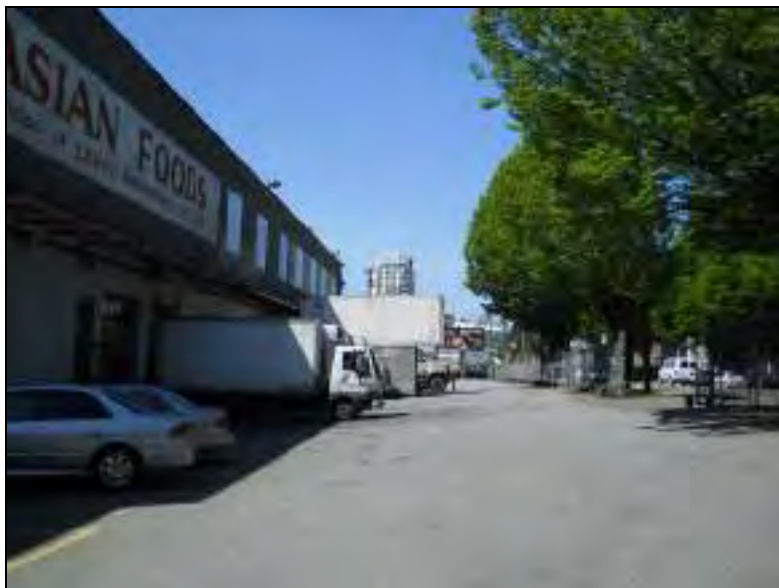
Photograph 4: The north portion of 456 Prior Street (looking west)
