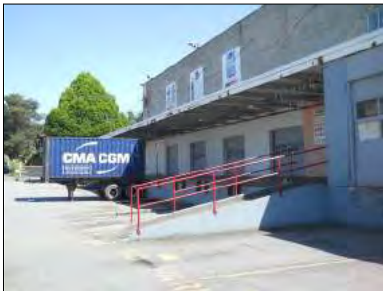
Photograph 6: The west portion of 456 Prior Street (looking northeast)
