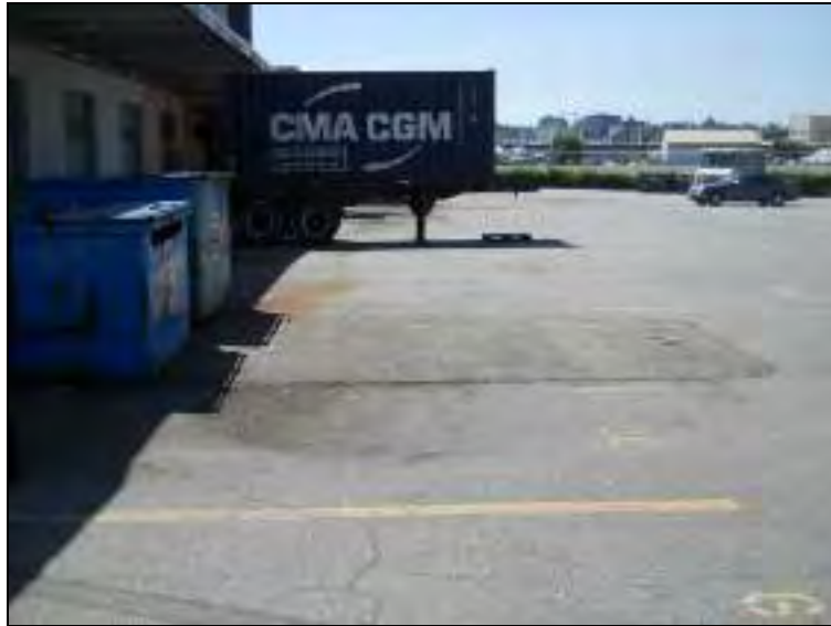
Photograph 7: The concrete pad on the northwest portion of 456 Prior Street (looking south)
