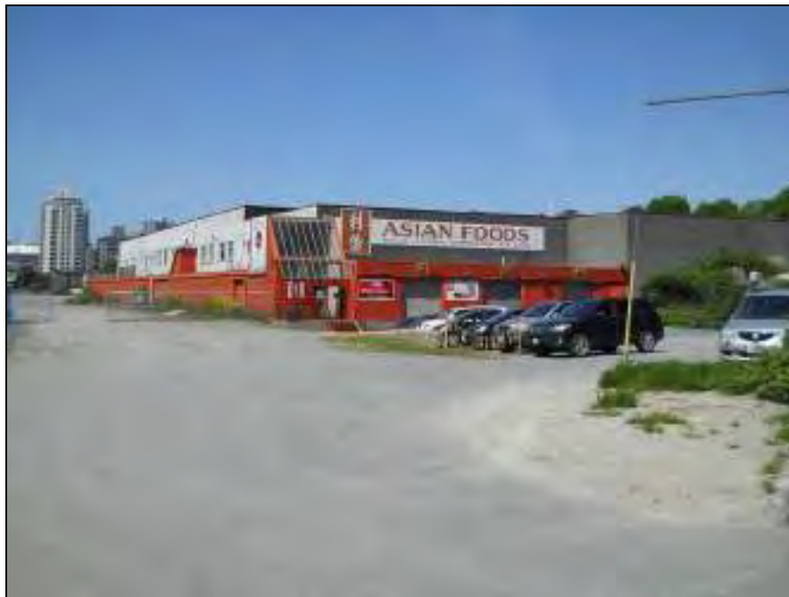
Photograph 2: The south portion of 456 Prior Street (looking northwest from 580 Malkin Street)
