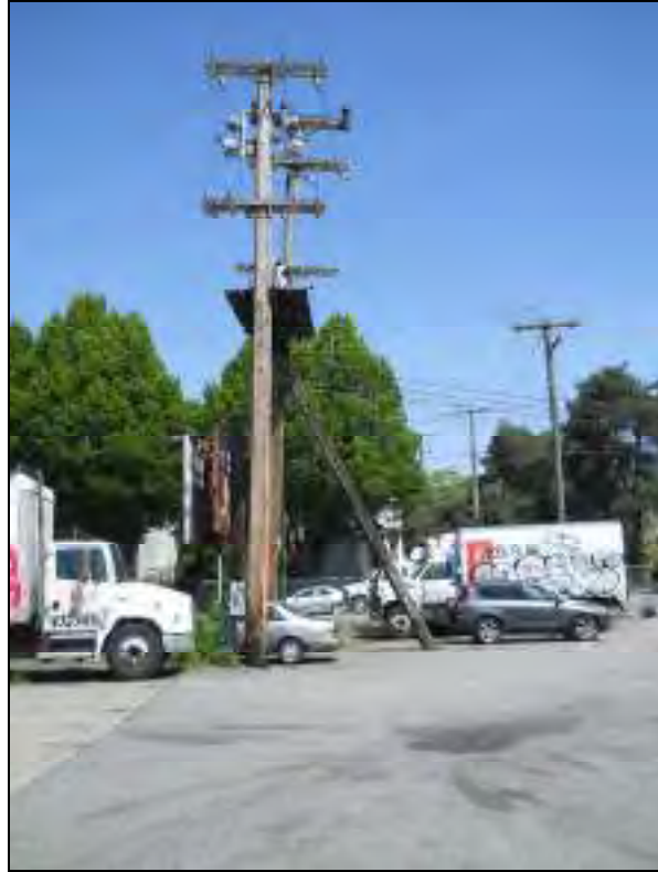
Photograph 5: The portion of the Site at 370 Prior Street (looking north)
