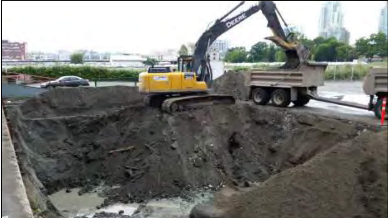
Photograph 1: View of the former UST area remedial excavation – looking southwest. June 02, 2015.
