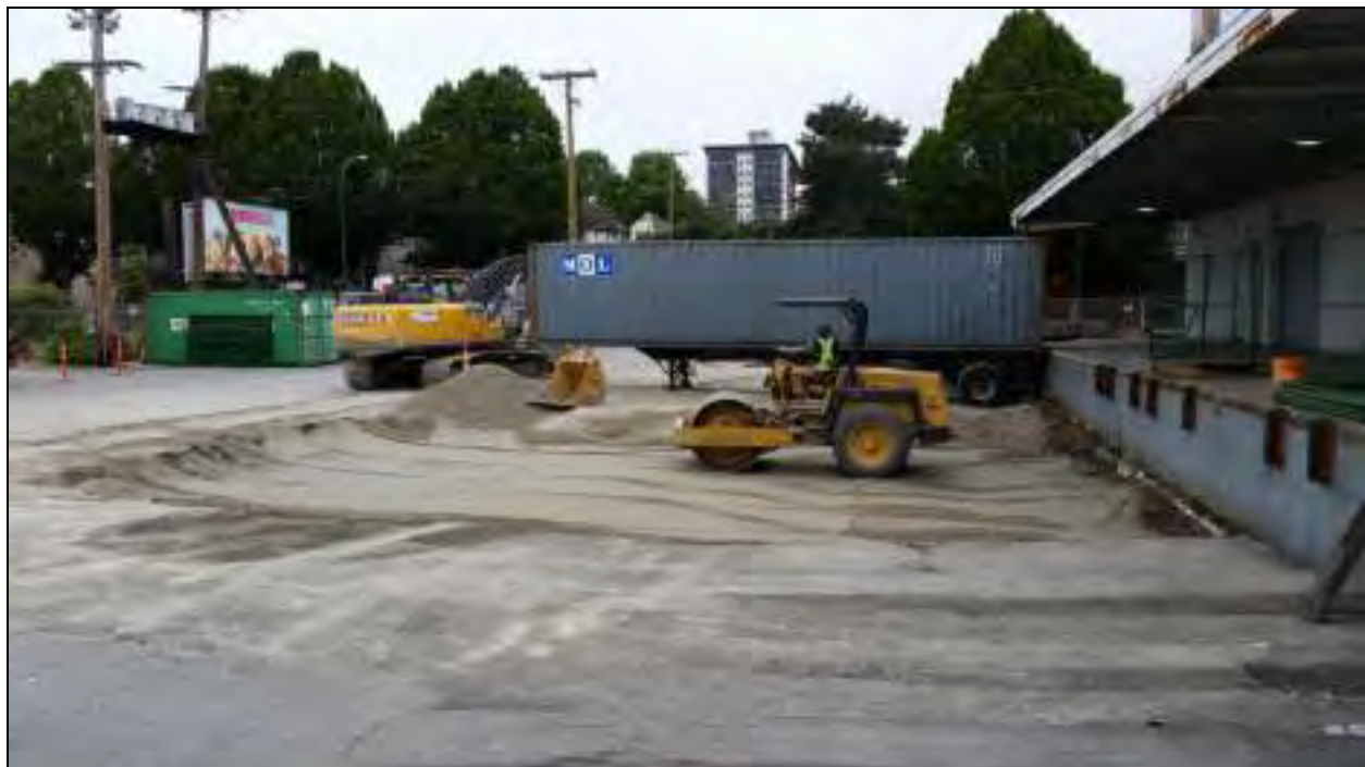
Photograph 4: View of the excavated area during backfilling activities – looking northwest. June 4, 2015.
