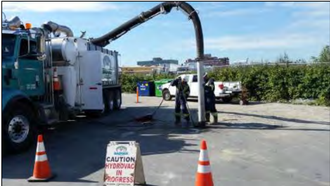
Photograph 3: Vacuum truck excavation north of CS15-14 (0.8) – looking south. June 25, 2015.
