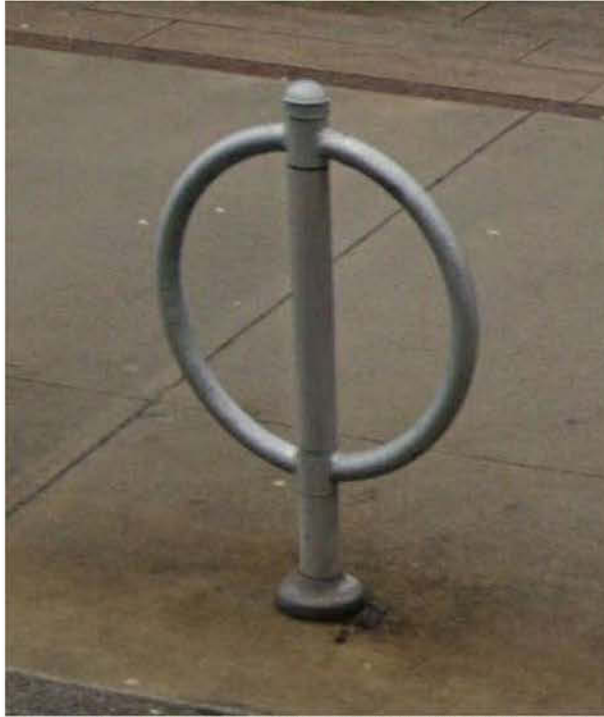
Figure 1 - Example of a “post and ring” bike rack retrofitted from a parking meter post
