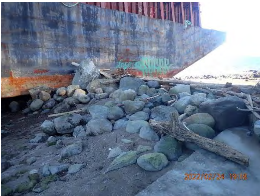
Photo 20 West Groyne - inshore end of groyne stepped due to barge, westward view.
