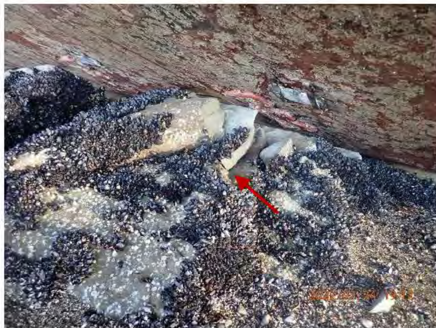
Photo 16 West Groyne - typical fractured rock under barge, west end.
