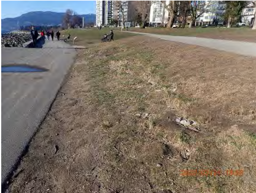
Photo 9 Between Paths - area of embankment erosion between west stairs and concrete pad to the east, approximately 10 m long.
