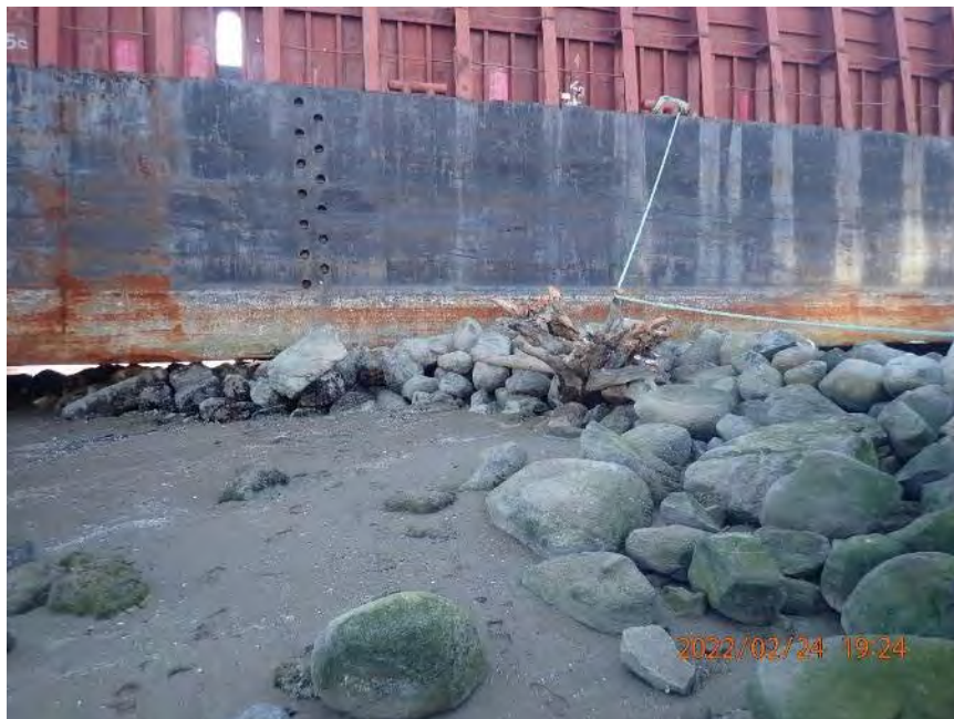
Photo 22 Centre Groyne - inshore end of groyne stepped due to barge, southward view.
