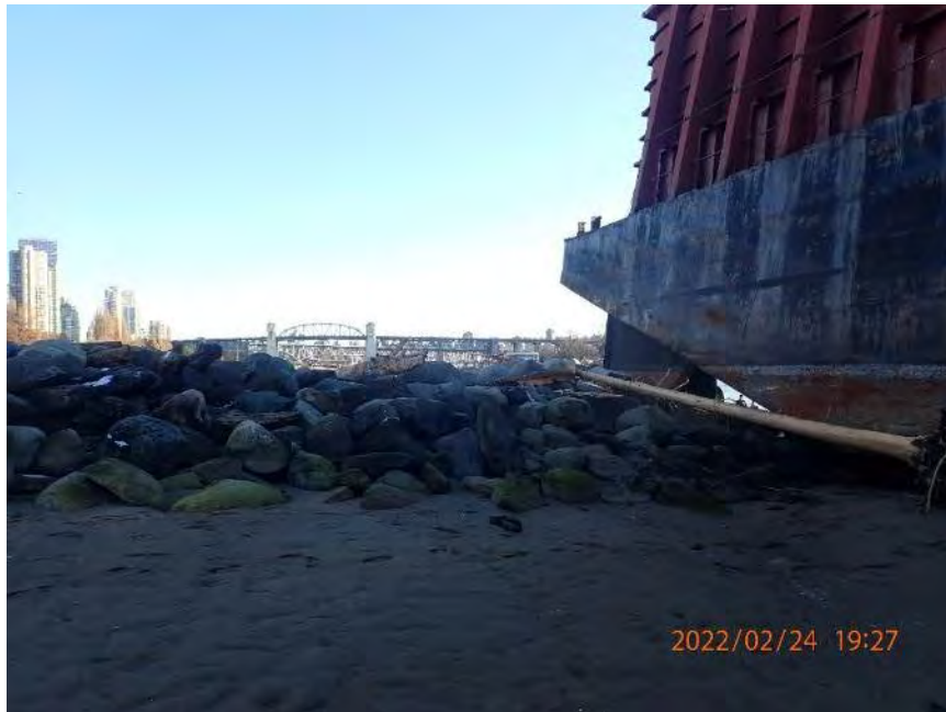
Photo 23 East Groyne - inshore end of groyne stepped due to barge, eastward view.
