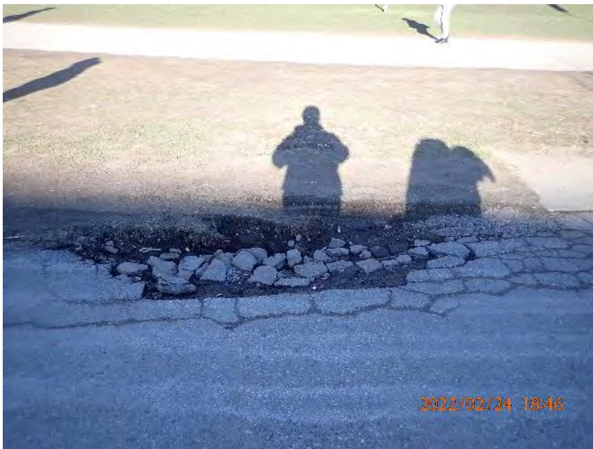
Photo 10 Offshore Path - asphalt failure along north edge of offshore path pavement, approximately 0.5 m wide by 1 m long.
