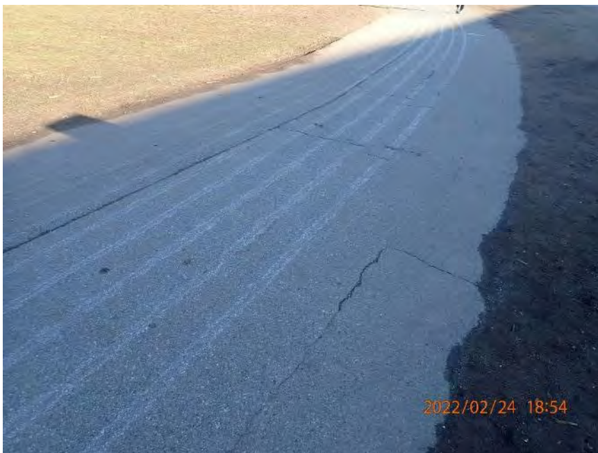
Photo 4 Inshore Path - typical localized asphalt cracking along path.
