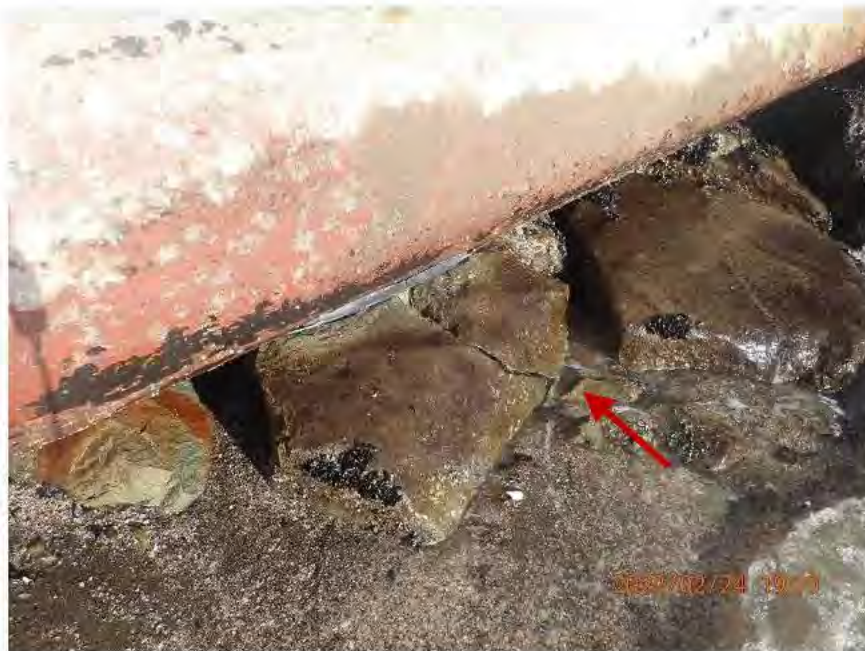
Photo 15 West Groyne - typical fractured rock under barge, offshore end.
