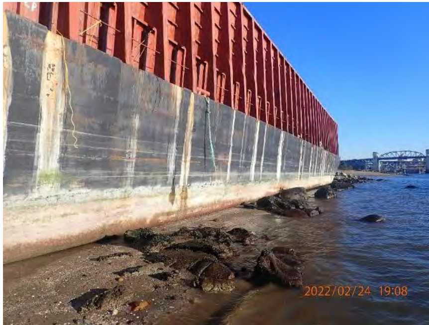
Photo 21 Centre Groyne - assumed offshore end of groyne demolished by barge, eastward view south of barge.
