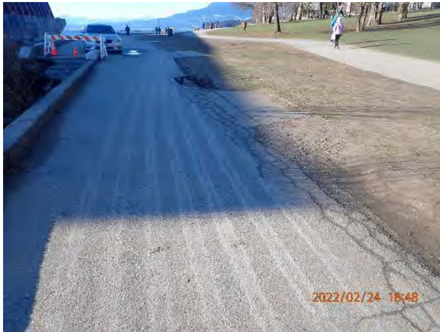
Photo 11 Offshore Path - cracking along north edge of offshore path pavement approximately 10 m long.
