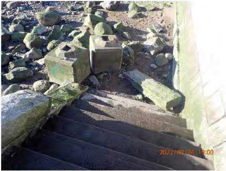
Photo 13 West Seawall Stairs – displaced capstone at bottom of stairs.
