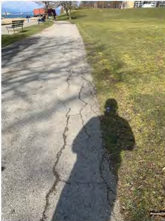
Photo 3: Path with subgrade failure
