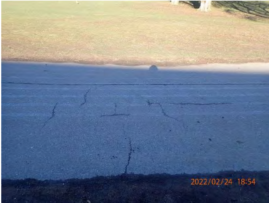
Photo 5 Inshore Path - typical localized asphalt cracking along path.
