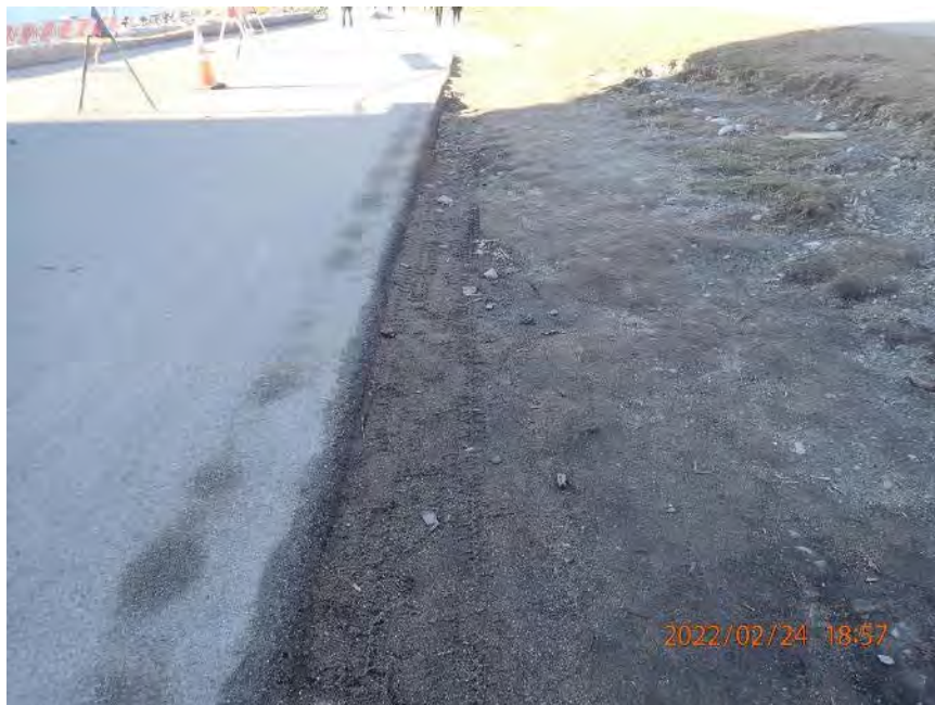
Photo 12 Offshore Path - scouring along north edge of offshore path approximately 10 m long.
