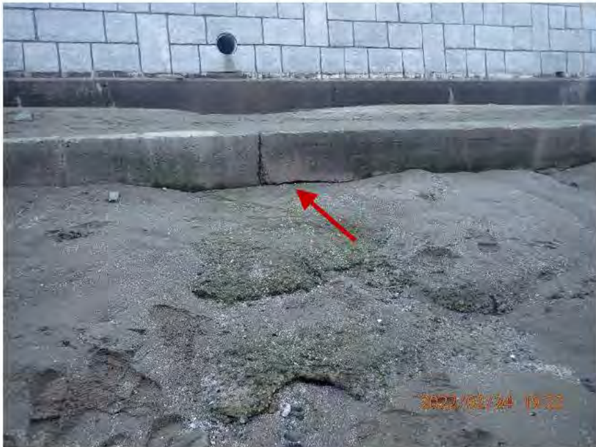
Photo 14 Seawall – toe of offshore end of wall beginning to undermine by approximately 25 mm between west and centre groyne.
