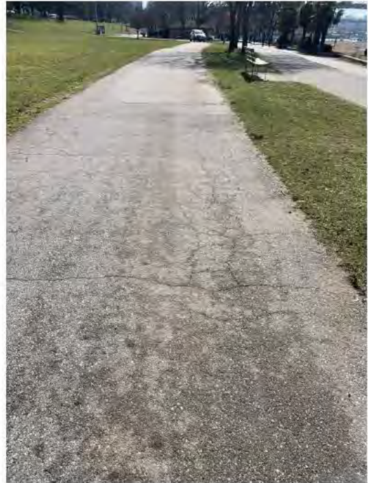
Photo 2: Path with subgrade failure
