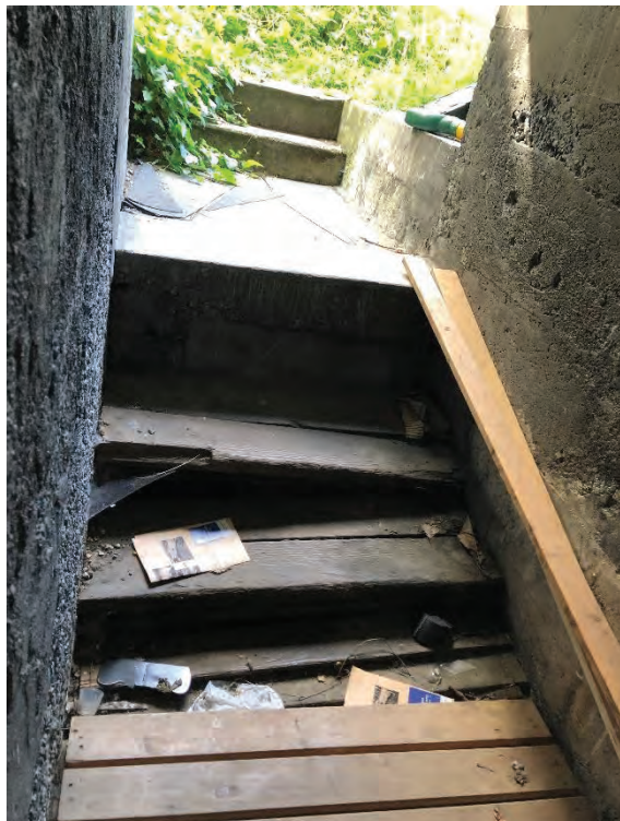
Basement access/egress stair out collapsed and step hazard
