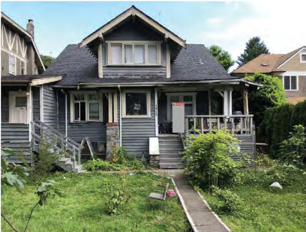
Front elevation-general rotting structure dilapidated building, rotted access stair boards/guards and roof falling pieces/collapsing hazard. Structural columns leaning and rotting support underside.
