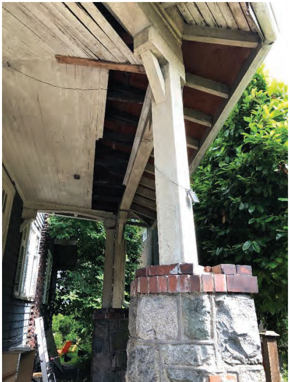
Another roof support post leaning & evidence of fallen soffit boards, brick work
