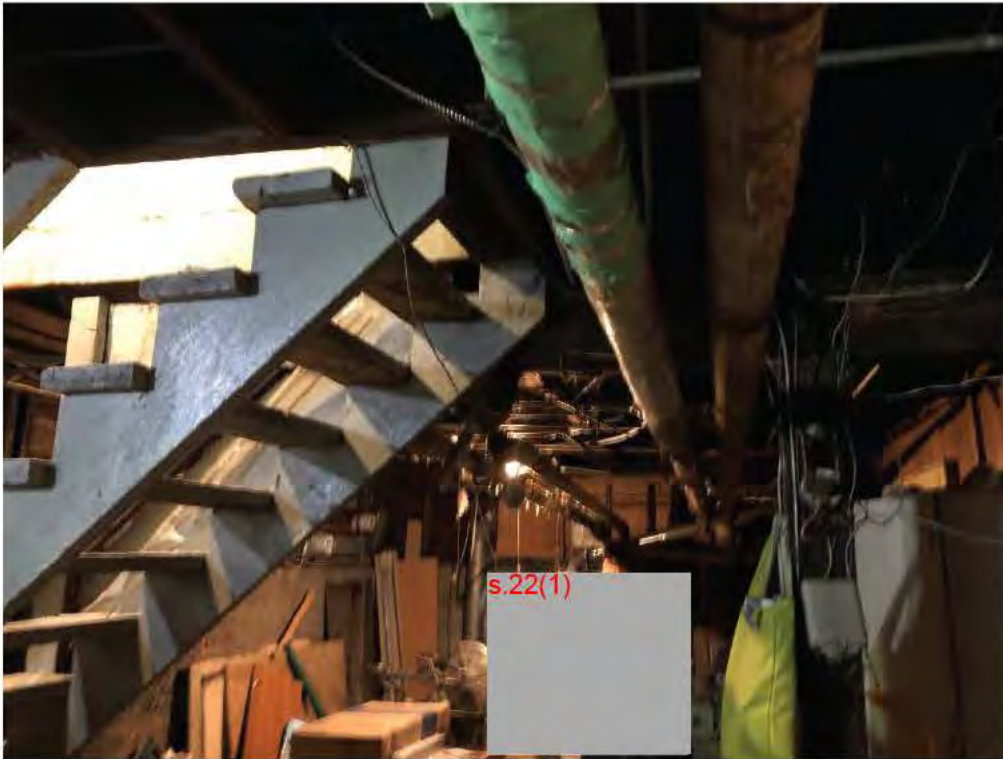
Basement clutter, no fire-separation as required, access and service fire hazard
