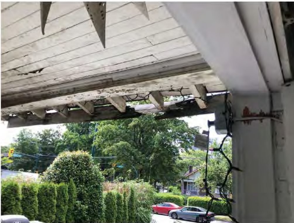
General rotted cladding/structure, roof fascia boards falling and gutters
