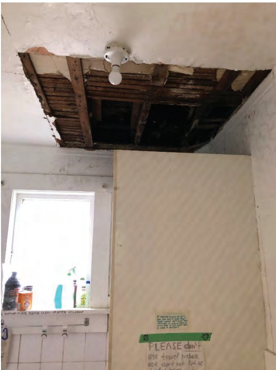
Main floor ceiling collapsed from leak above where the upper washroom is no longer working
