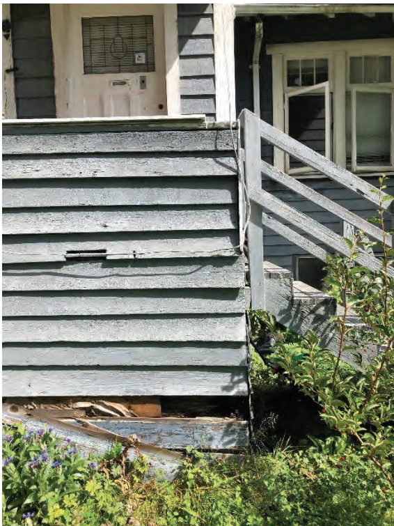
Rotted bearing support under roof post
