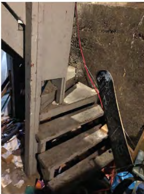
Unsafe access/egress stair basement to the main floor
