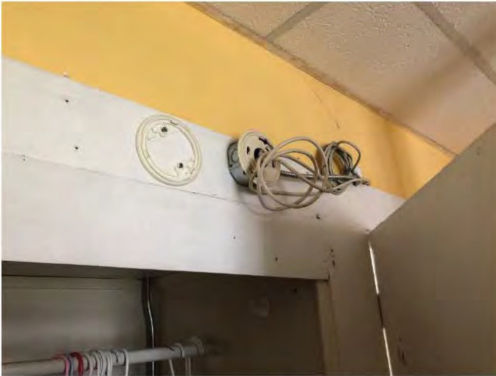
Noncomplying smoke alarms and exposed wiring typical throughout - safety hazard
