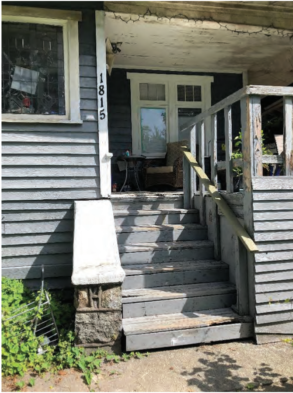
Front entry stair/treads rotted and crumbling-access/egress safety hazard
