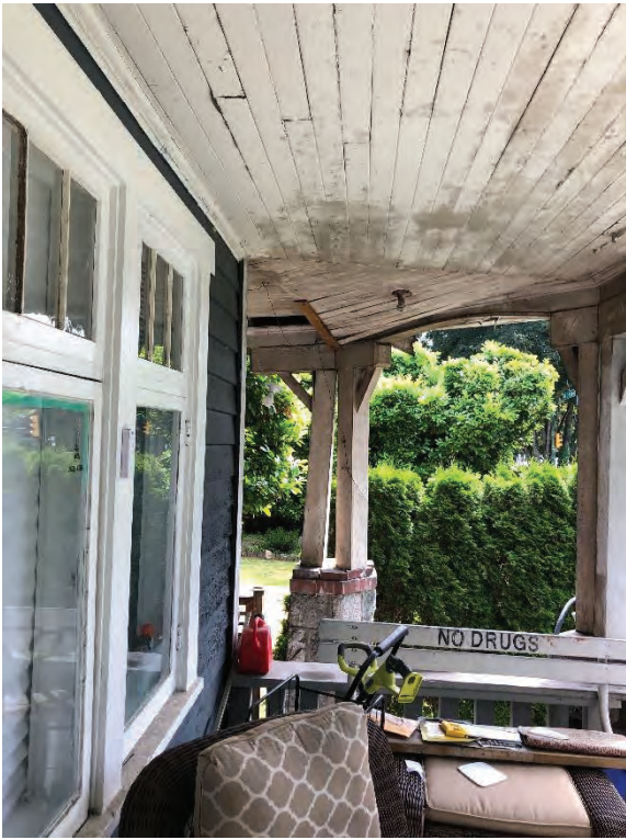
Front porch roof support posts leaning/collapsing and roof pieces falling
