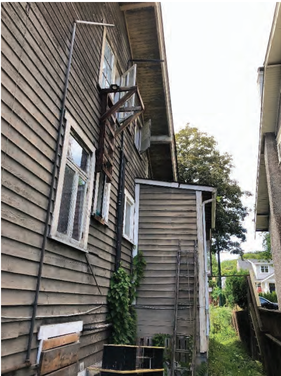
Unsafe fire exit ladder from the top floor & debris below
