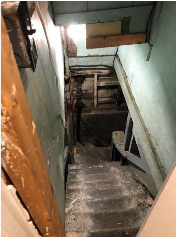
Main floor looking down unsafe stair design and access to basement & no handrails, non-complying guard
