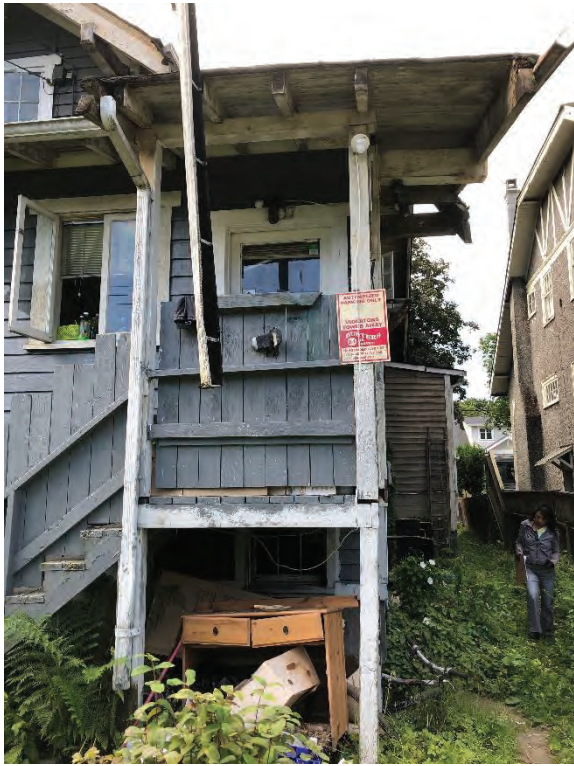
Rear main floor access/egress porch roof support post leaning/collapsing & rafter support fascia board missing & gutter hanging etc-unsafe
