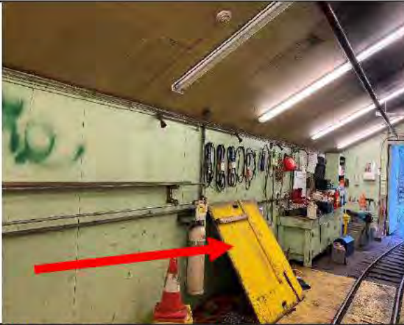
Photo 5: Yellow Paint on Wooden Floor Panels. Lead Based Paint.
