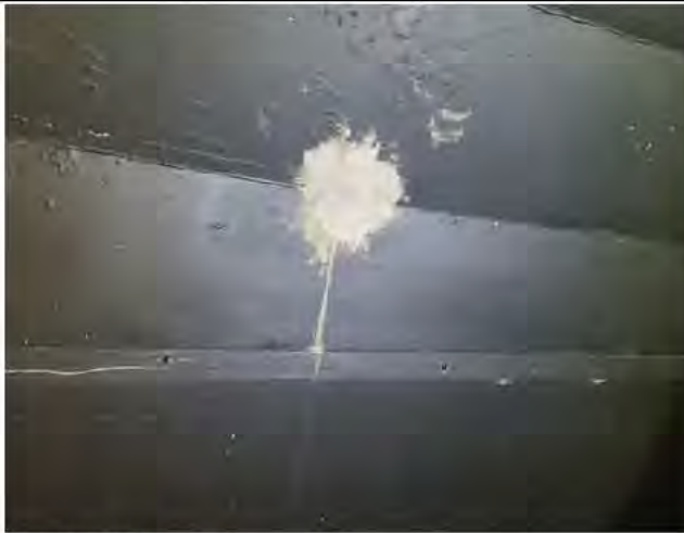
Previous epoxy repair
