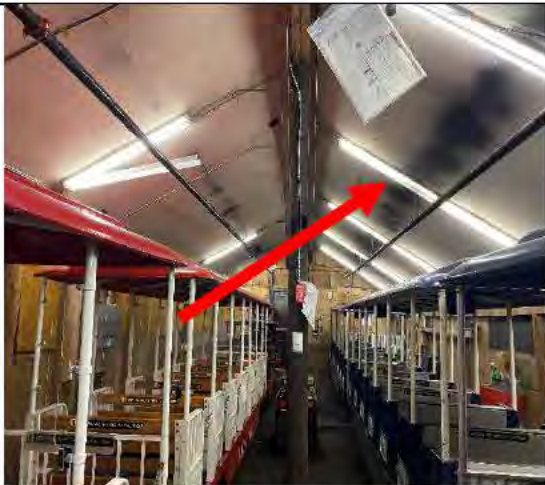
Photo 3: Fluorescent Tubes on Ceiling. Containing Mercury.
