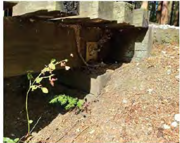
19 - West Abutment - debris accumulation (2021 )
