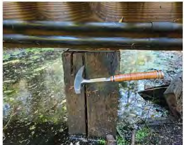
17 - Pier 1, North Post, north face - 50% section loss (2022 )
