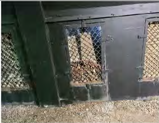
Debris accumulation in wall opening
