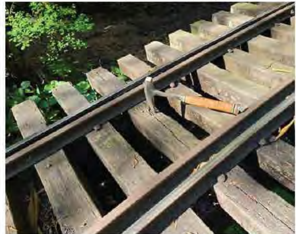
16 - Cross-ties - checks and weathering (2022 )
