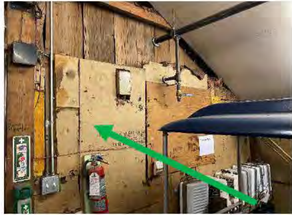
Photo 6: Tar Like Material on Fiberglass Wall Panels. Non-Asbestos Containing.
