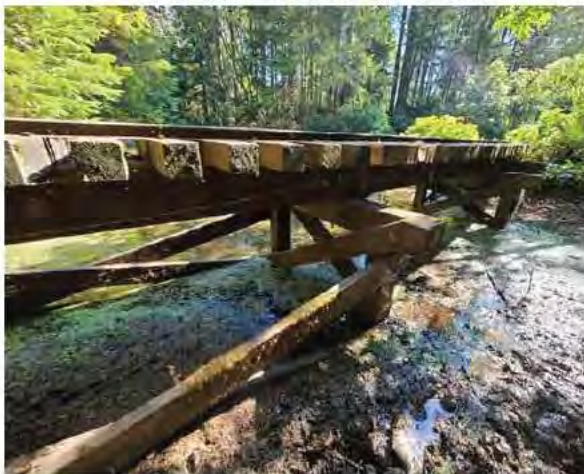
20 - South Elevation - algae growth typical (2022 )
