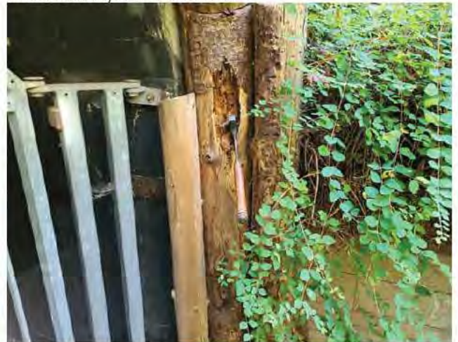
Tunnel entrance, timber fascia - decay and insect infestation
