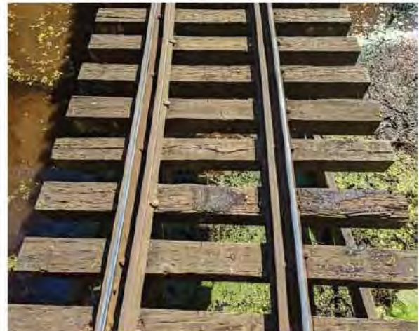
17 - Cross-ties - weathering, and checks (2022 )
