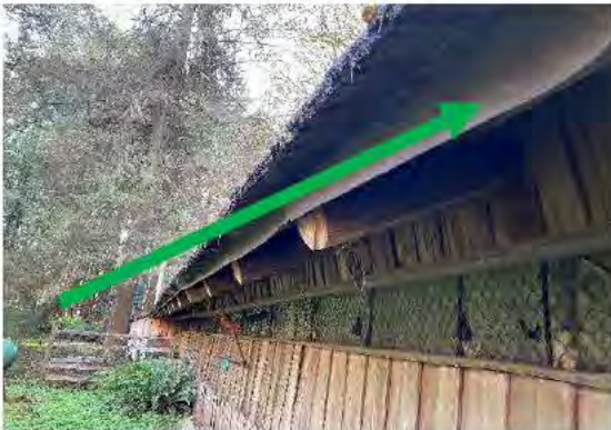
Photo 7: Black Insulation Paper under Wooden Shingles Roof. Non-Asbestos Containing.
