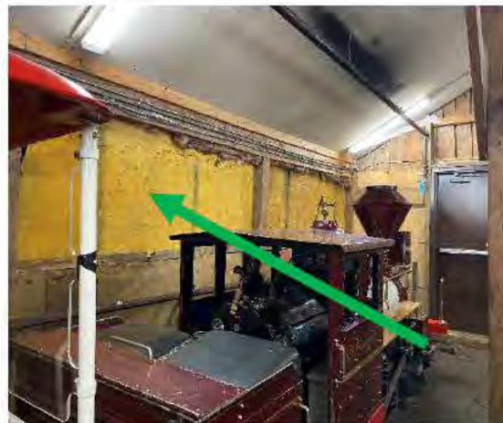
Photo 4: Tar Like Material on Fiberglass Wall Panels. Non-Asbestos Containing.
