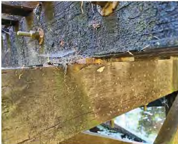
16 - Bearing Plate - corrosion (2022 )
