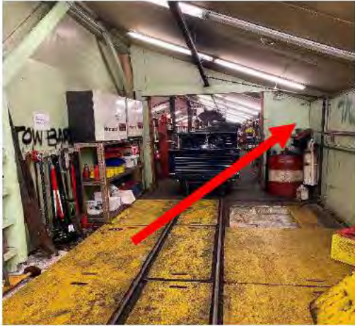
Photo 1: Green Paint on Wooden Walls - Pitt Area Only. Lead Based Paint.
