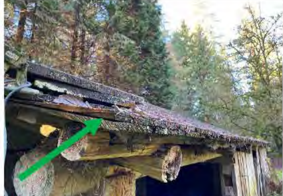
Photo 8: Black Insulation Paper under Wooden Shingles Roof. Non-Asbestos Containing.
