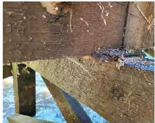
21 - Bearing plate - corrosion flaking (2022 )
