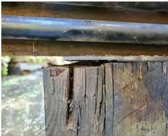
16 - Pier 1, North Post - settled section partially non-bearing and sister to bearing post (2022 )
