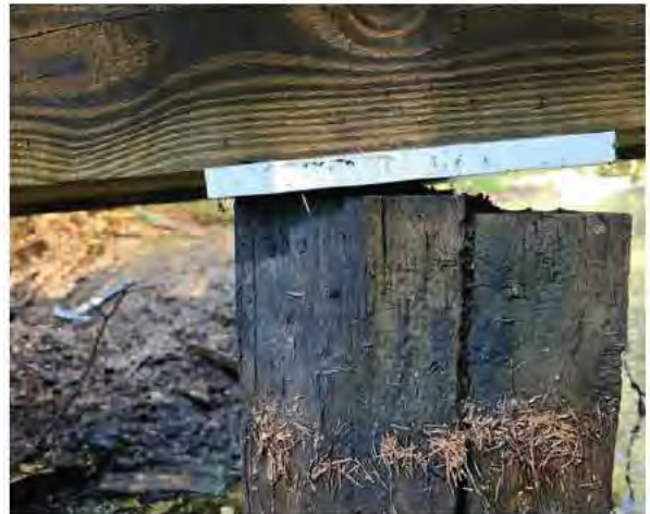
15 - Pier 1, South Post - settled section non-bearing and sistered to bearing post (2022 )
