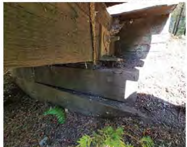
12 - West Abutment - misalignment of headwall (2022 )
