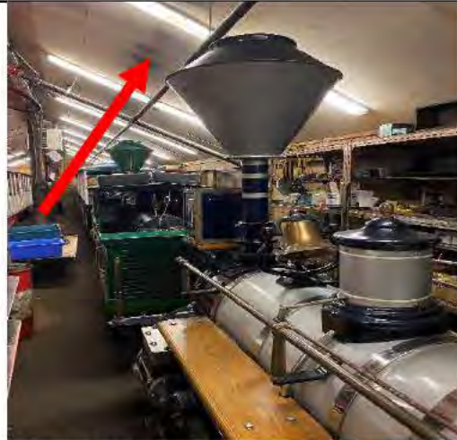
Photo 2: Cream Paint on Wooden Ceiling - Throughout Building. Lead Based Paint.
