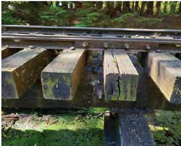
15 - Cross-ties - end splits typical (2022 )
