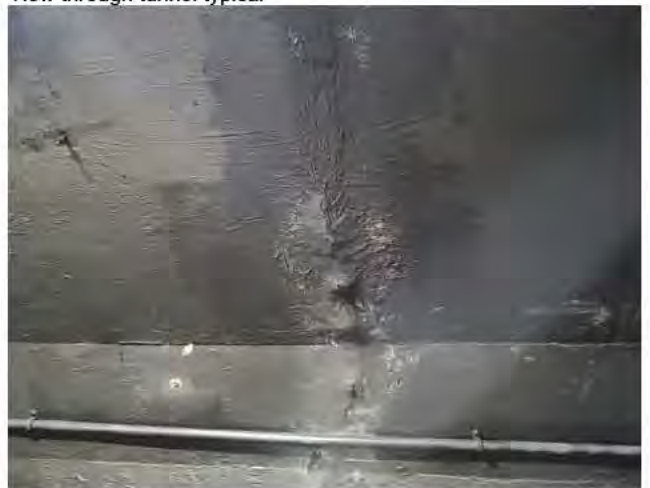
Roof section joint typical
