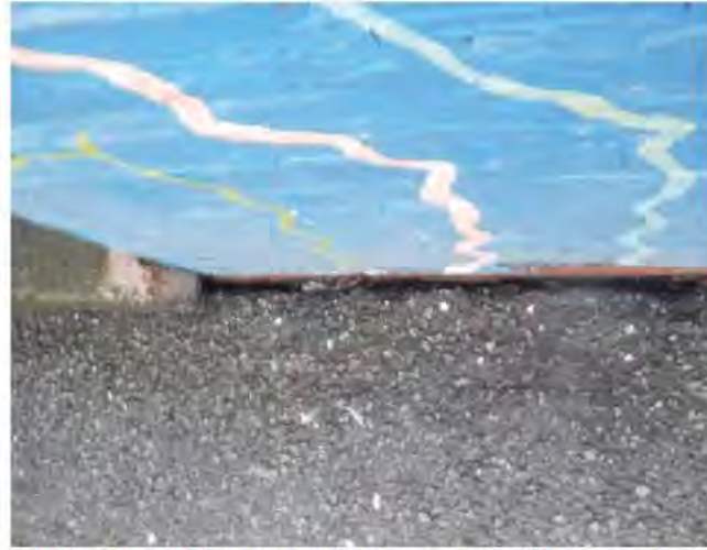
Photo 20: February 6, 2020 east side of lane east of Development Site
