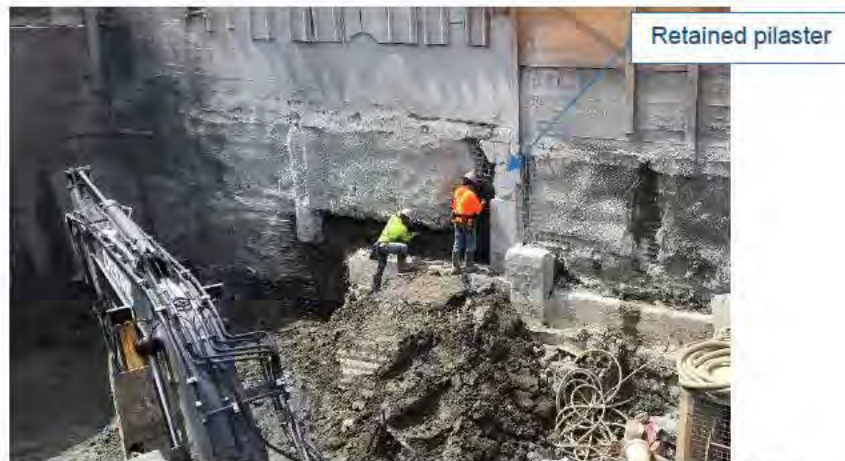
Photo 6: 3-day panel excavation sequence not followed, May 9, 2019
