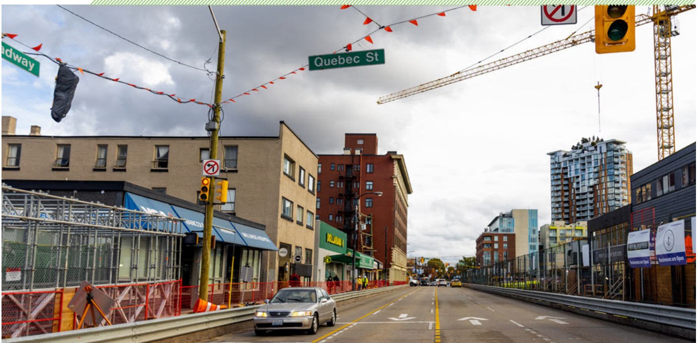
Source: Broadway Subway Project
