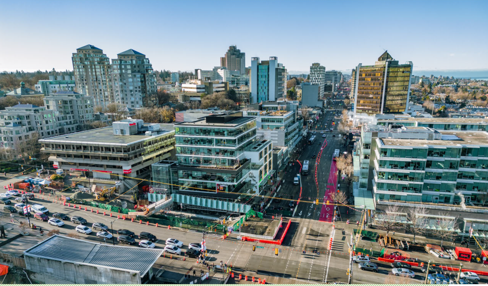
Source: Broadway Subway Project
