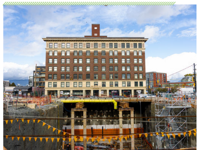
Source: Broadway Subway Project
