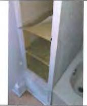
Photo 8: Asbestos-containing sheet vinyl flooring on shelving in staff washroom
