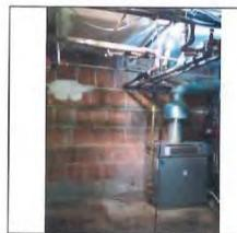
Photo 5: Asbestos-containing penetration mastic in boiler room
