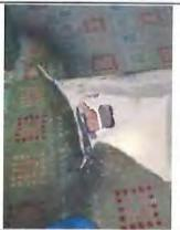
Photo 7: Asbestos-containing sheet flooring under carpet in Lockers room
