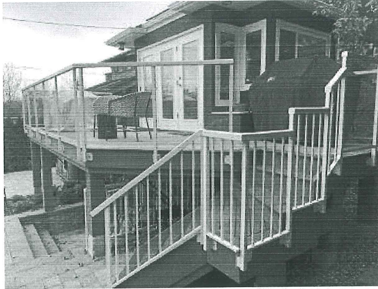
Upgraded Deck (2022) High Construction Standard
