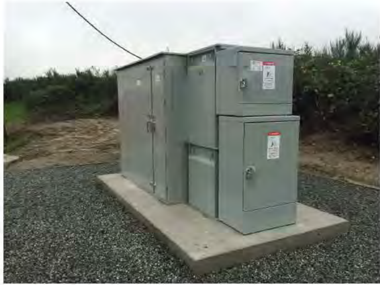
TYPICAL OUTDOOR UNIT SUBSTATION INCLUDING PRIMARY SWITCH GEAR & TRANSFORMER - 1 N.T.S.
