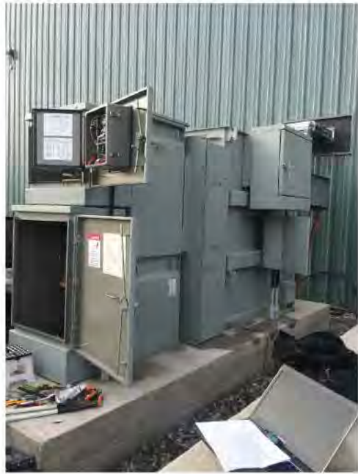
TYPICAL OUTDOOR UNIT SUBSTATION INCLUDING PRIMARY SWITCH GEAR & TRANSFORMER - 2 N.T.S.
