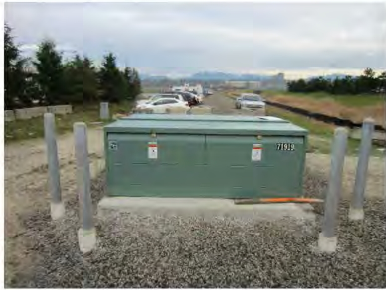
TYPICAL OUTDOOR VISTA TYPE PRIMARY SWITCHGEAR N.T.S.
