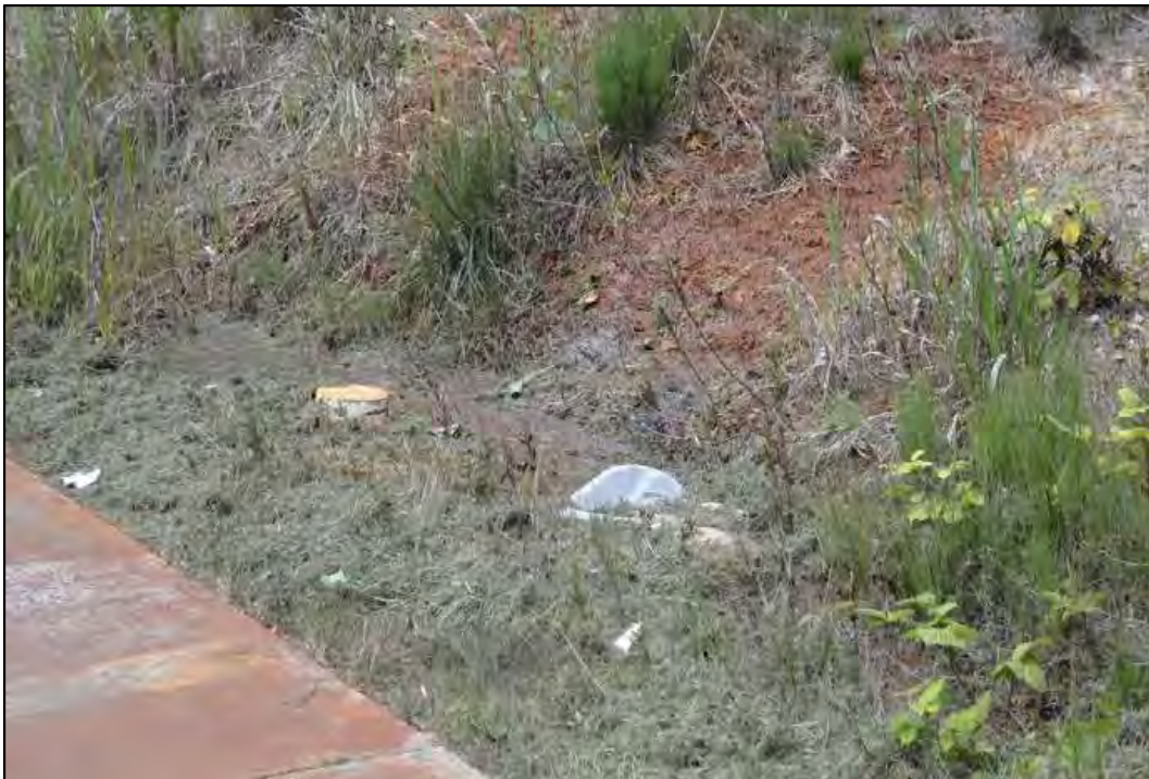
PHOTO 24: Close-up of iron staining (Seep D) and one of 2 x 6" diameter capped PVC piping. (June 12, 2014)
