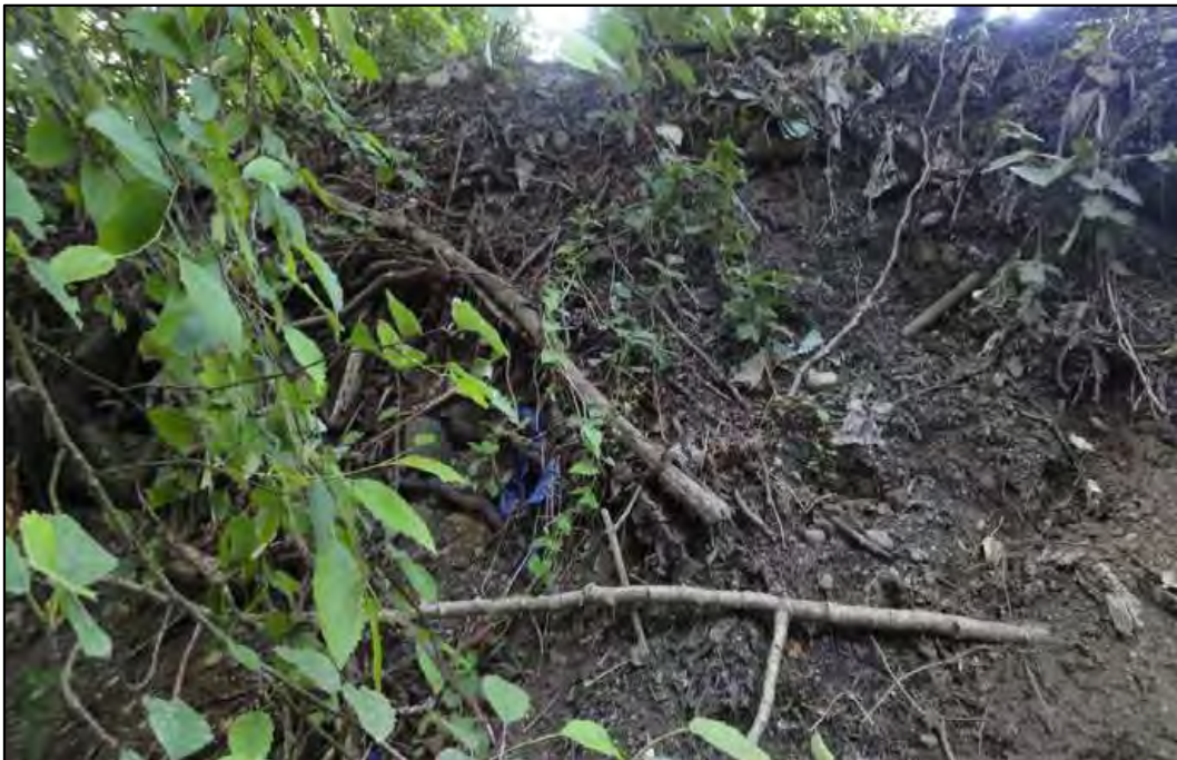
PHOTO 13: Close-up of debris Photo 11 creek area. (June 12, 2014)
