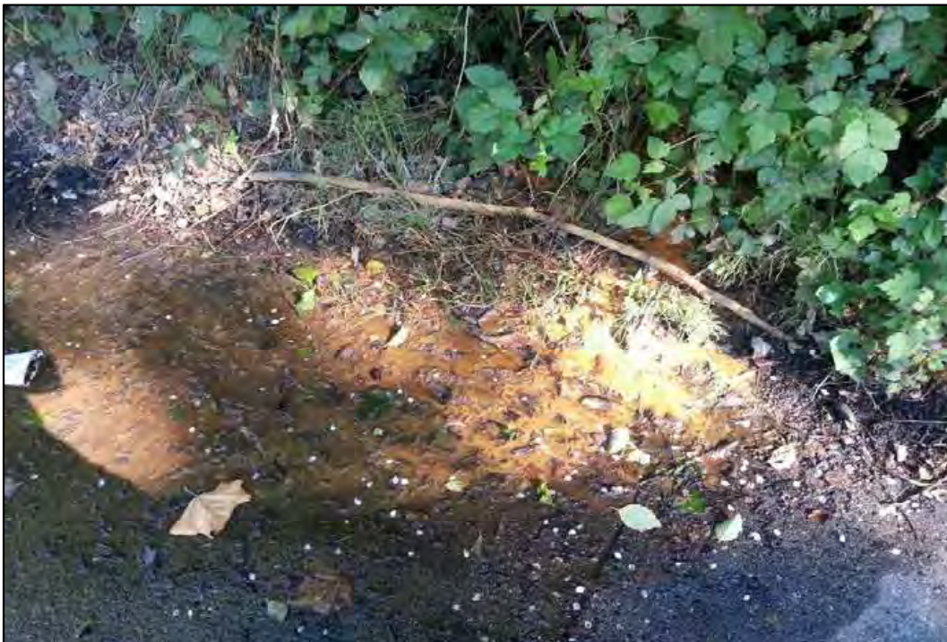
PHOTO 35: Seep onto sidewalk on Matheson Avenue (Close-up) (June 30, 2014)
