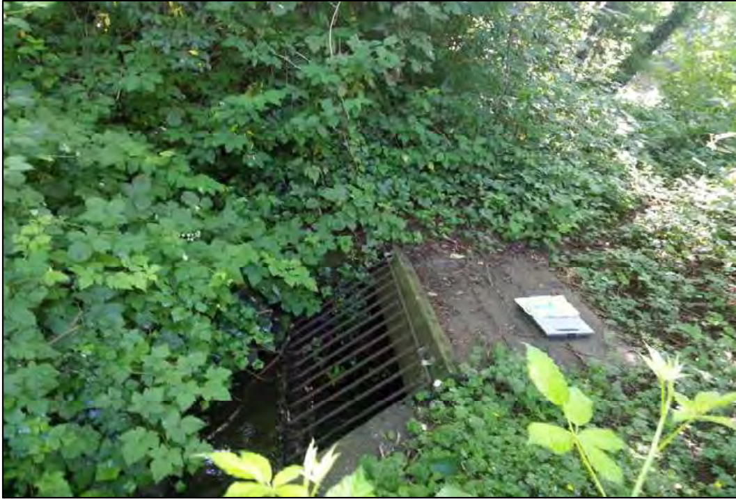
PHOTO 36: Storm drain for outfall from New Kinross Creek. (June 30, 2014)
