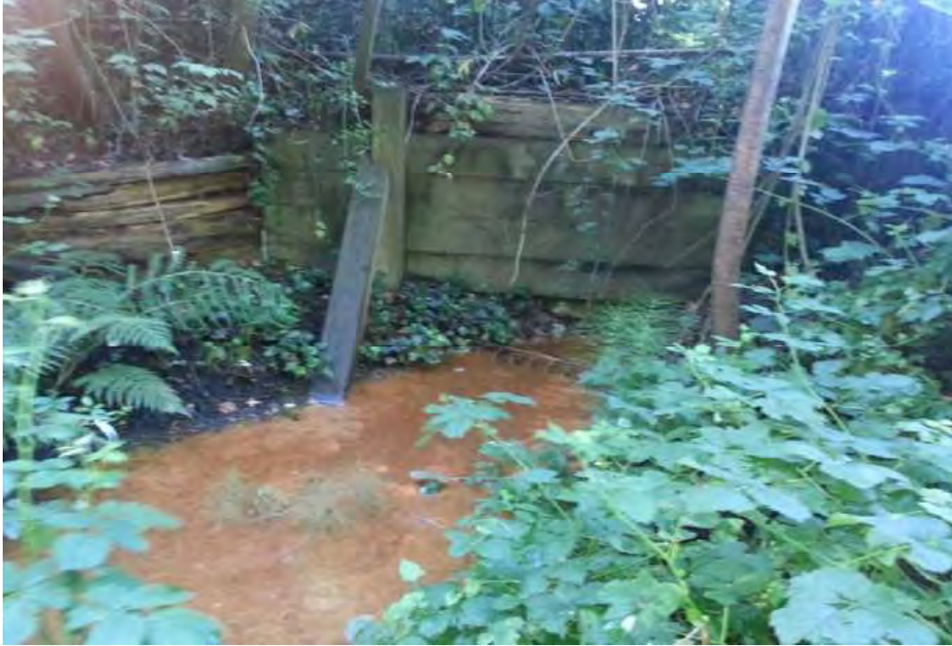
PHOTO 40: Termination of iron-laden water (wooden barricade and metallic grate). (June 30, 2014)
