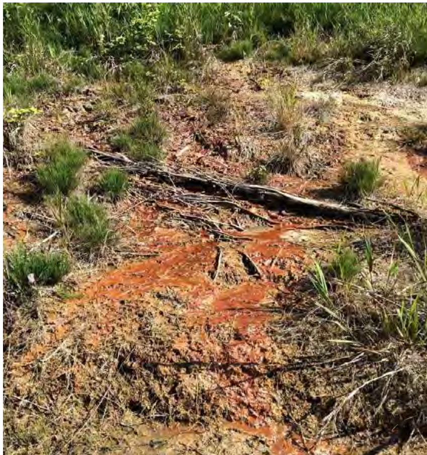
Photo 2: Seepage from 2 m above base of toe along south slope 100 m (approx.) east of Kerr St.
