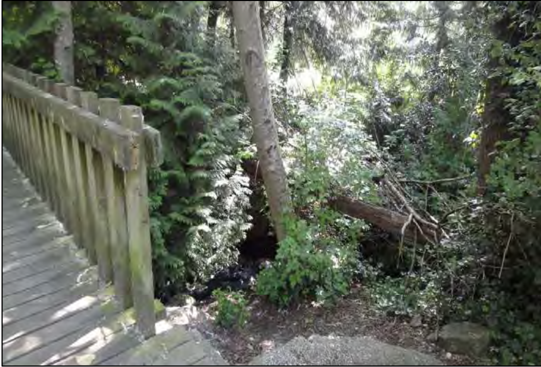
PHOTO 14: Bridge crossing New Kinross Creek, looking southeast and downstream. (June 12, 2014)
