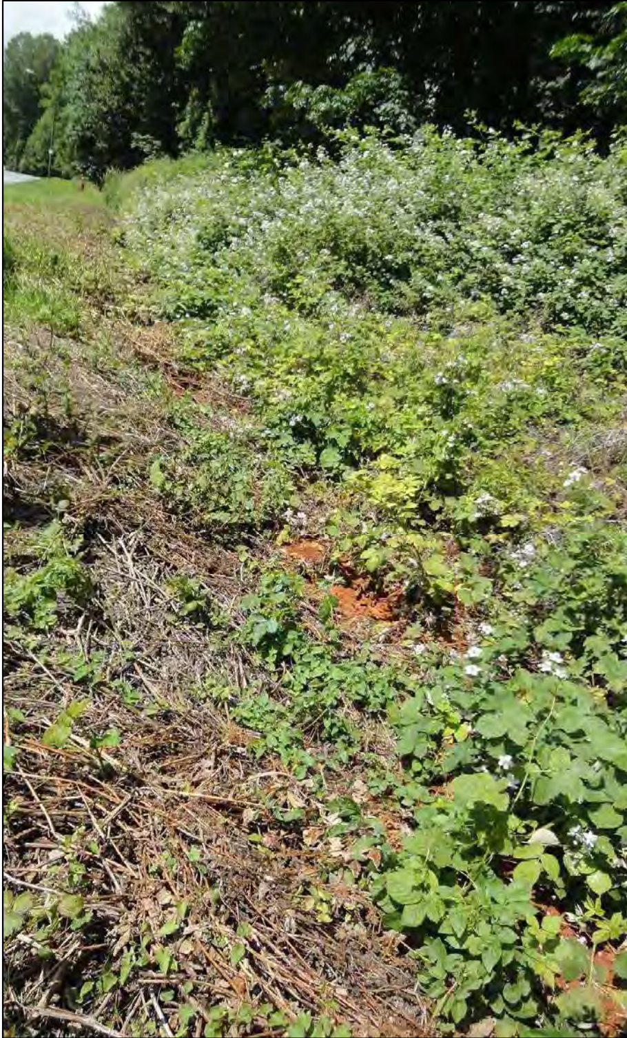
PHOTO 20: Visible iron staining (Seep B) along Marine drive in small swale at toe of slope. (June 12, 2014)
