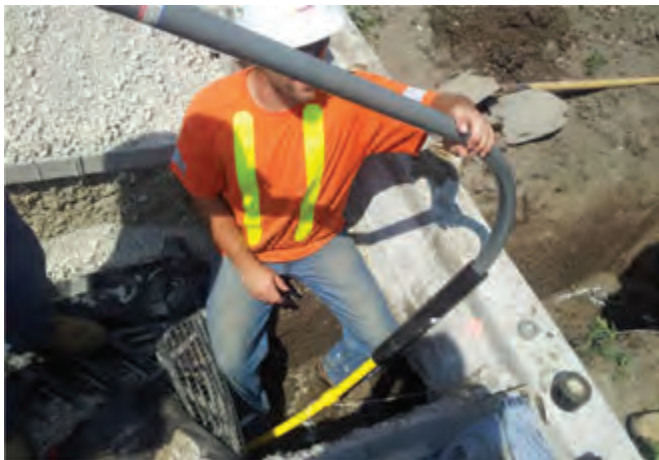
Riser is attached and pulled through.
