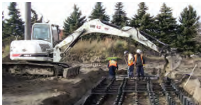
Soil cell trench filled with soil.
