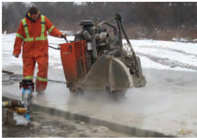
Sawcutting concrete pavement.
