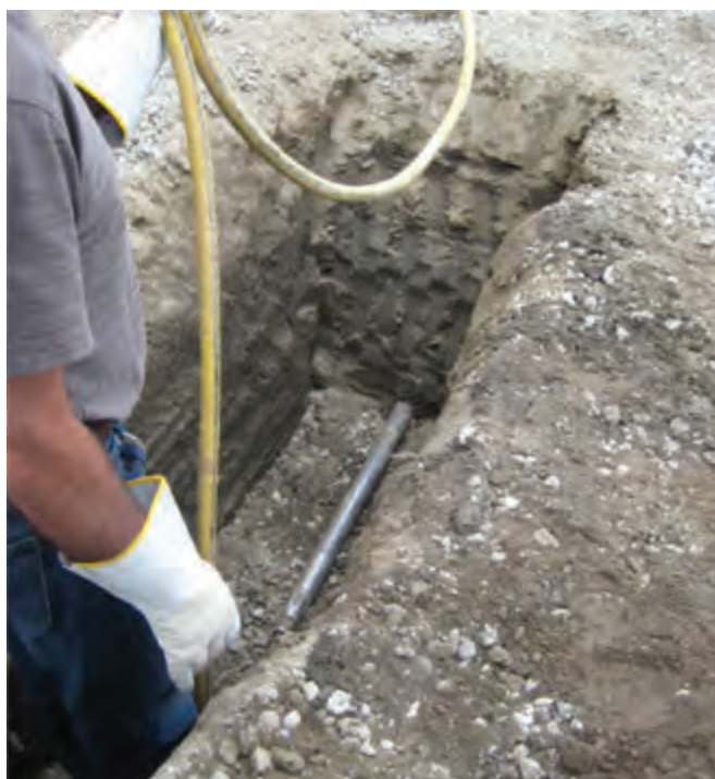
After false start on imaginary building end, torpedo is reset at road end.
