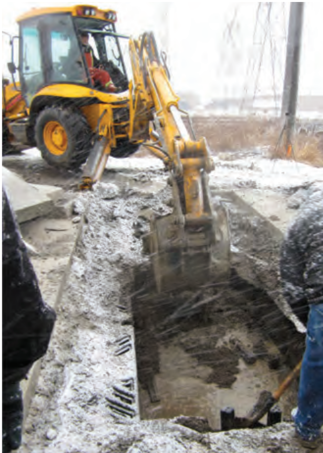
Mechanical removal of soil cells.
