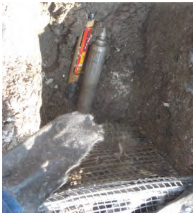
Torpedo emerges through growing medium and cell decks on the imaginary building side.
