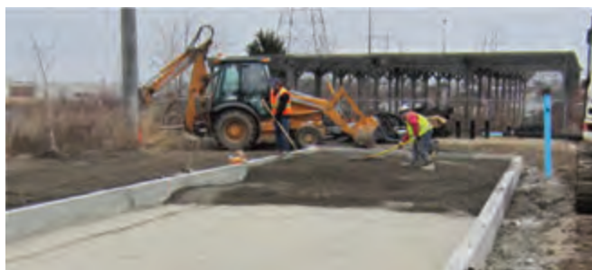
Backfill installation on top of deck.
