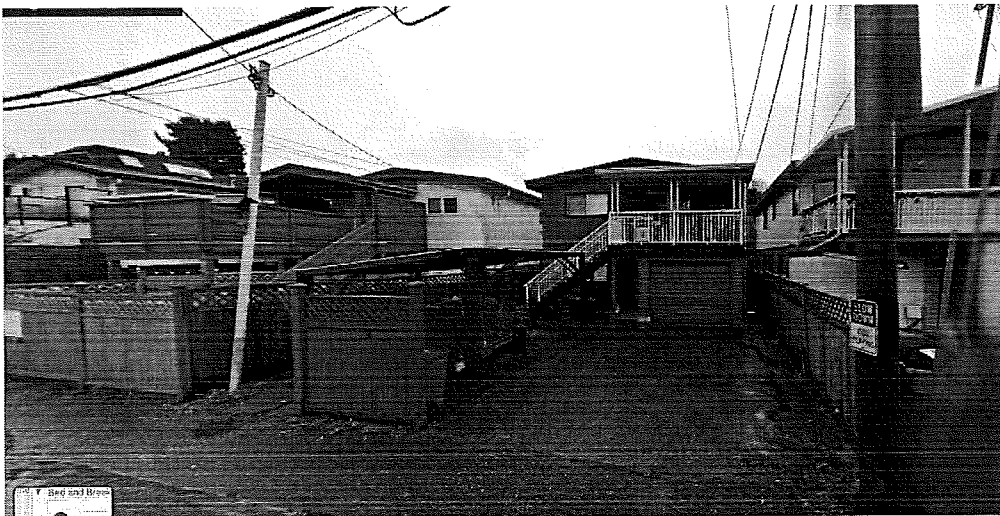
Figure 1 - Rear of 5560 Chester Street. Red Enclosure was removed in 2021.
