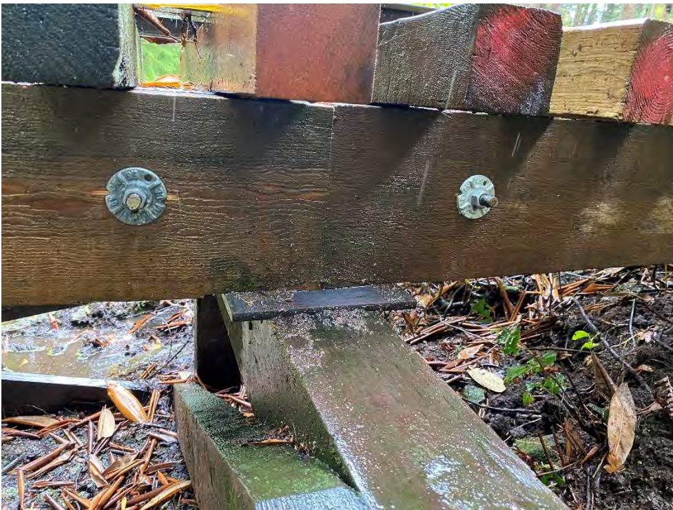
Photograph 2: Stringer sistering at pier bent No. 9 (B-45).
