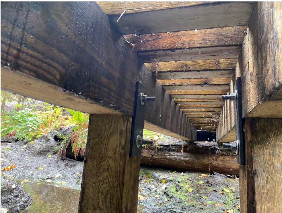
Photograph 6: Columns connection plates, looking northeast (B-46).
