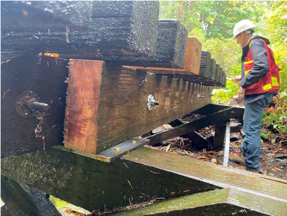
Photograph 2: Stringer sistering at pier bent No. 9 (B-45).
