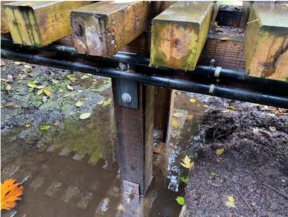
Photograph 6: Columns connection plates, looking northeast (B-46).
