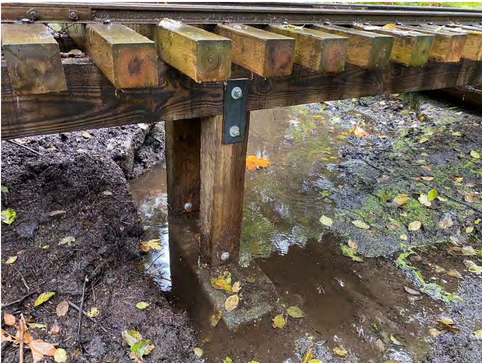
Photograph 4: Southeast column on concrete footing (B-46).
