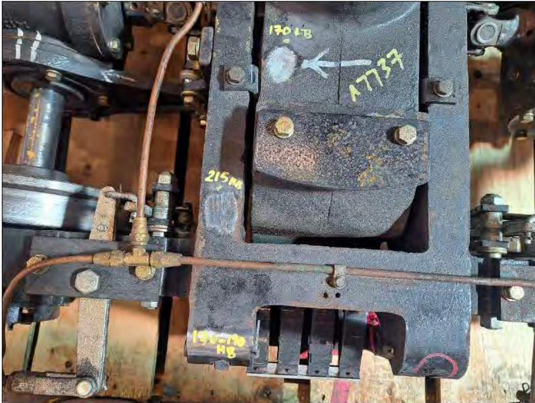
Figure 16 Area polished to identify any weld repairs – none found.
