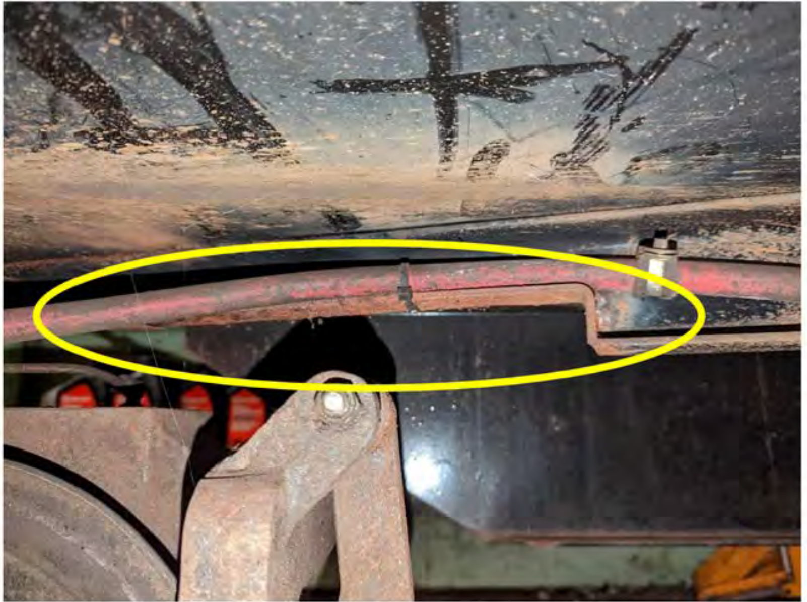
Figure 29: Frame modifications & poor weld quality
