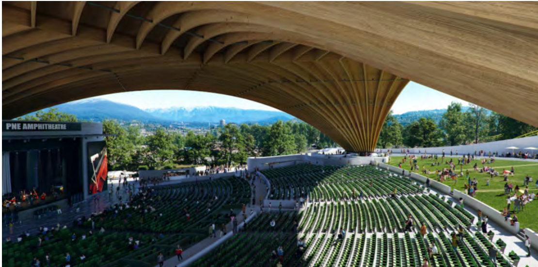
Figure 6 - The mass timber roof envelops the audience area, strategically limiting sound spread, improving acoustic performance, and allowing for distributed and targeted sound reinforcement. (Image by Mir courtesy of Pacific National Exhibition [PNE])
