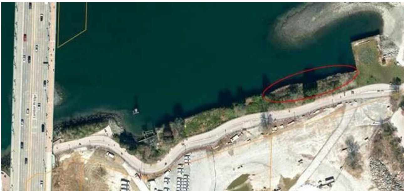
Fig. 1 – Cambie sheetpile wall: approximate area of concern shown in red
