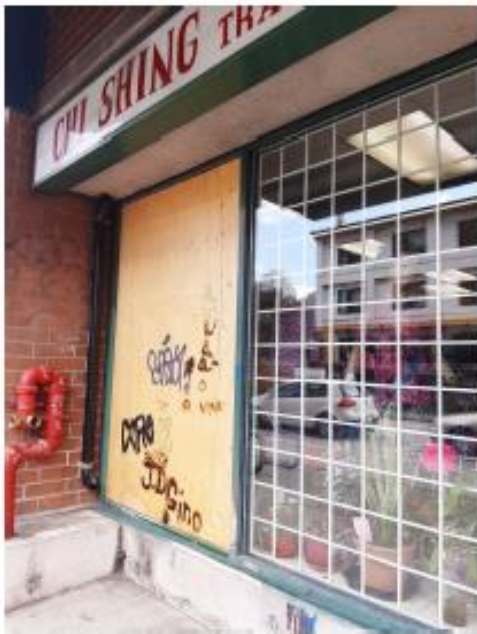
Picture 3: Exterior of Chi Shing before glass replacement
