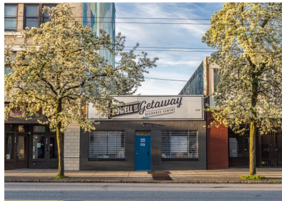
Picture 10: Exterior of the site after renovation
