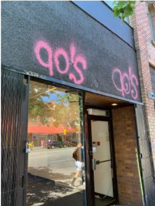
Picture 1. Exterior of THIS Gallery before shutter gate installation
