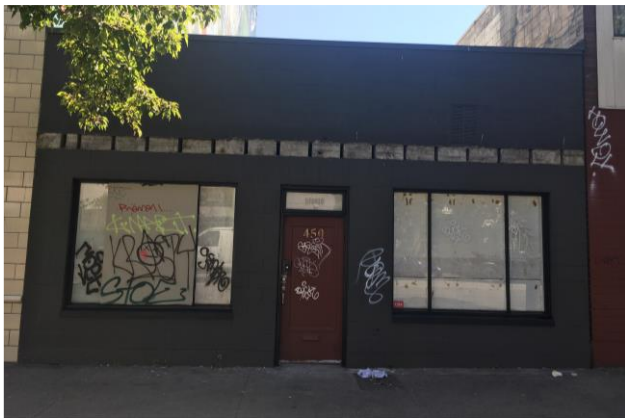
Picture 9: Exterior of the site before renovation
