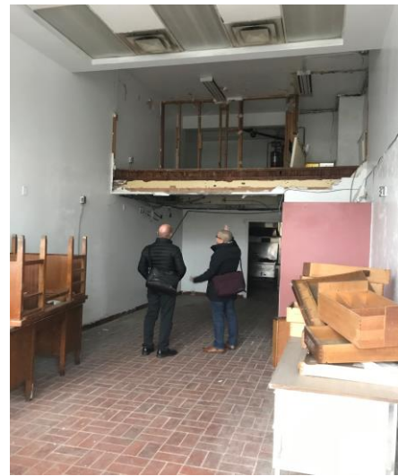
Picture 8: Interior of the site during renovation
