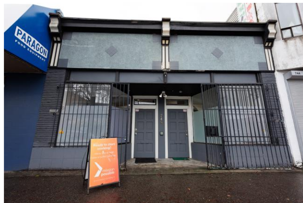
Picture 14: Exterior of the site after renovation
