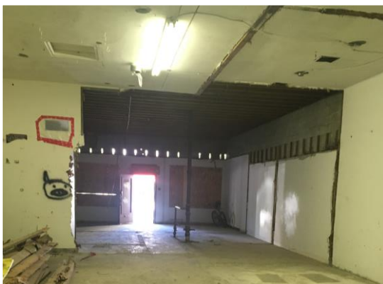
Picture 11: Interior of the site before renovation
