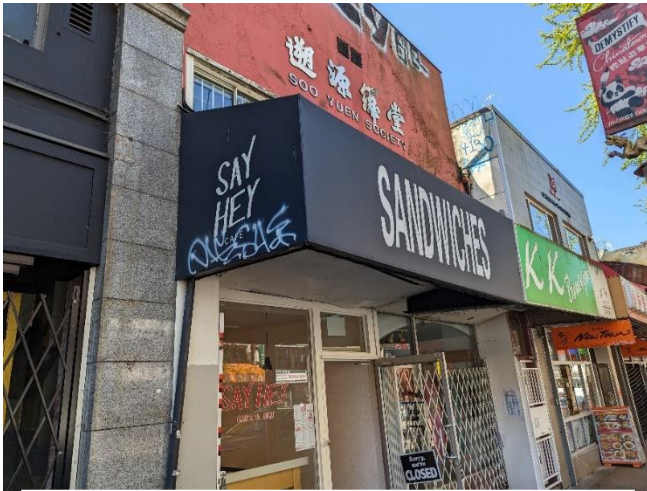
Picture 5: Exterior of Say Hey Café before the awning replacement.
