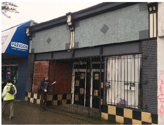
Picture 13: Exterior of the site before renovation
