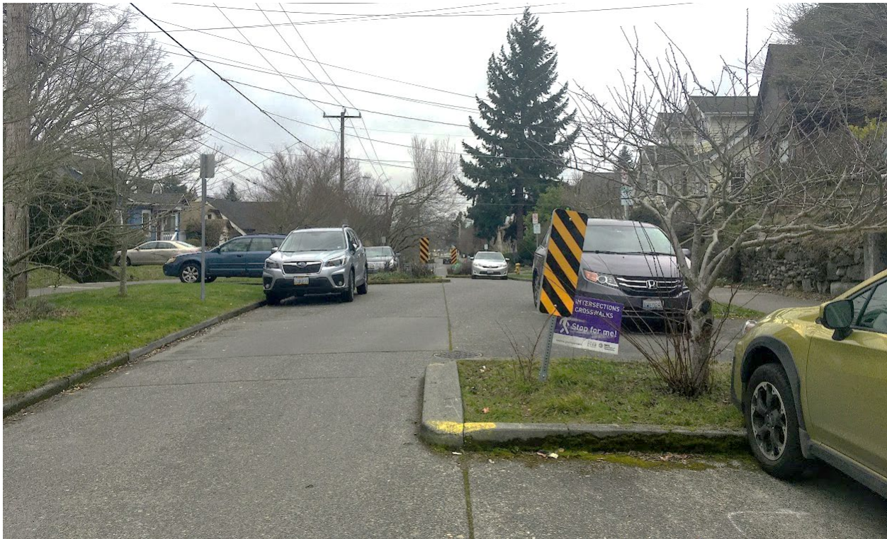
Figure A.6: Example of a chicane on a local street in Seattle, Washington
