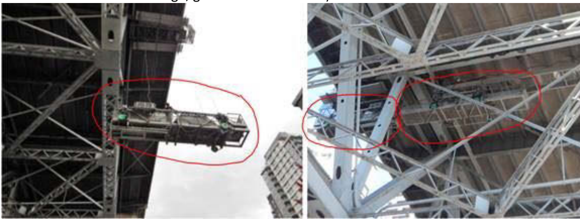
Figures 5 & 6 – Gantry units being used by City crews
