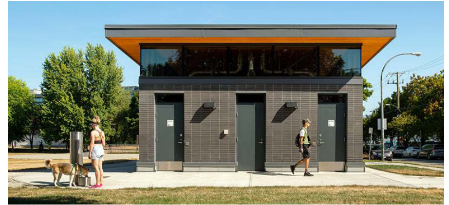
China Creek North Park Washrooms & Pump House
