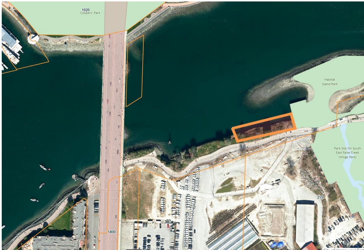
Figure 1 – approximate location of the Cambie sheet pile wall and Crowe St outfall (highlighted in orange)
