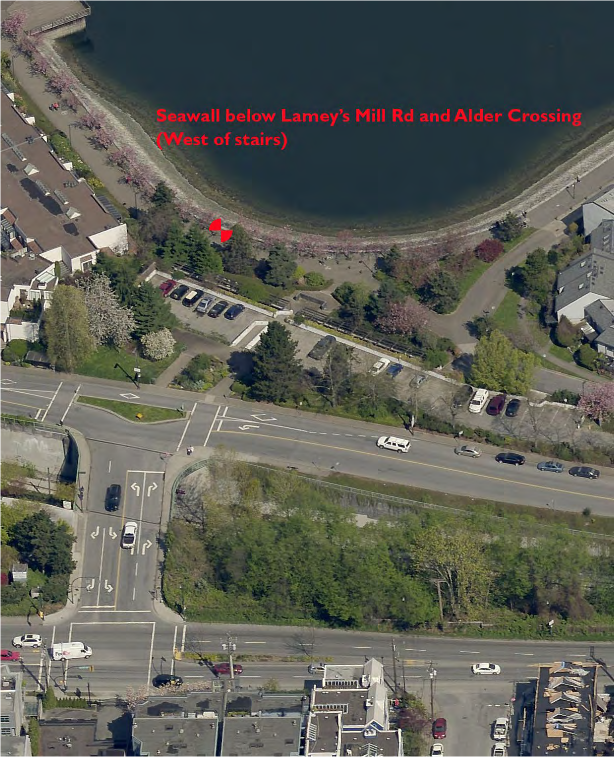
'A' View Point - Seawall below Lamey's Mill Road and Alder Crossing
