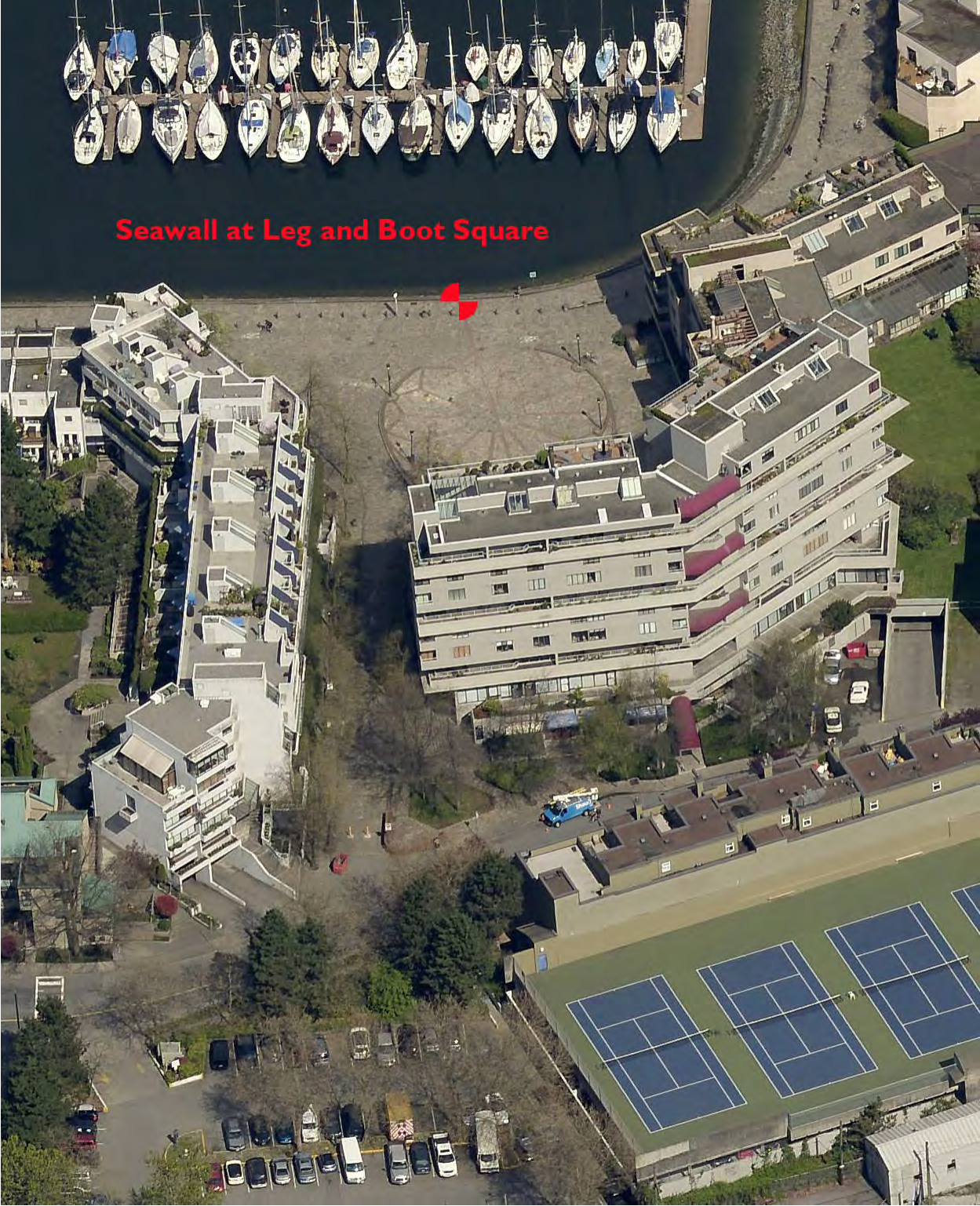
'D' View Point - Seawall at Leg and Boot Square
