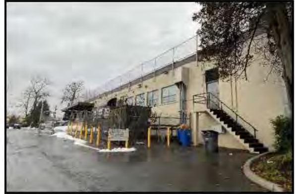
LOOKING WEST FROM KASLO STREET REAR OF SITE
