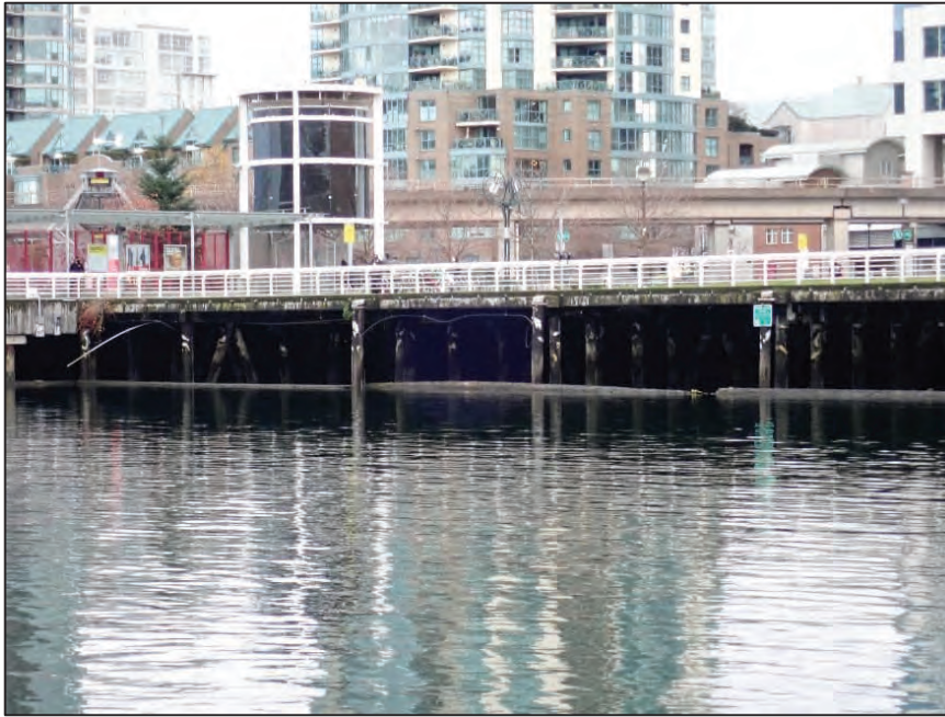
Photo 3-3 Typical View of Fendering System
