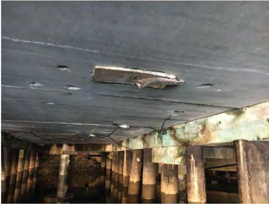
Photograph No.13: Previously installed formwork failing at Panel No. 5 between Bent Nos 23 and 24.
