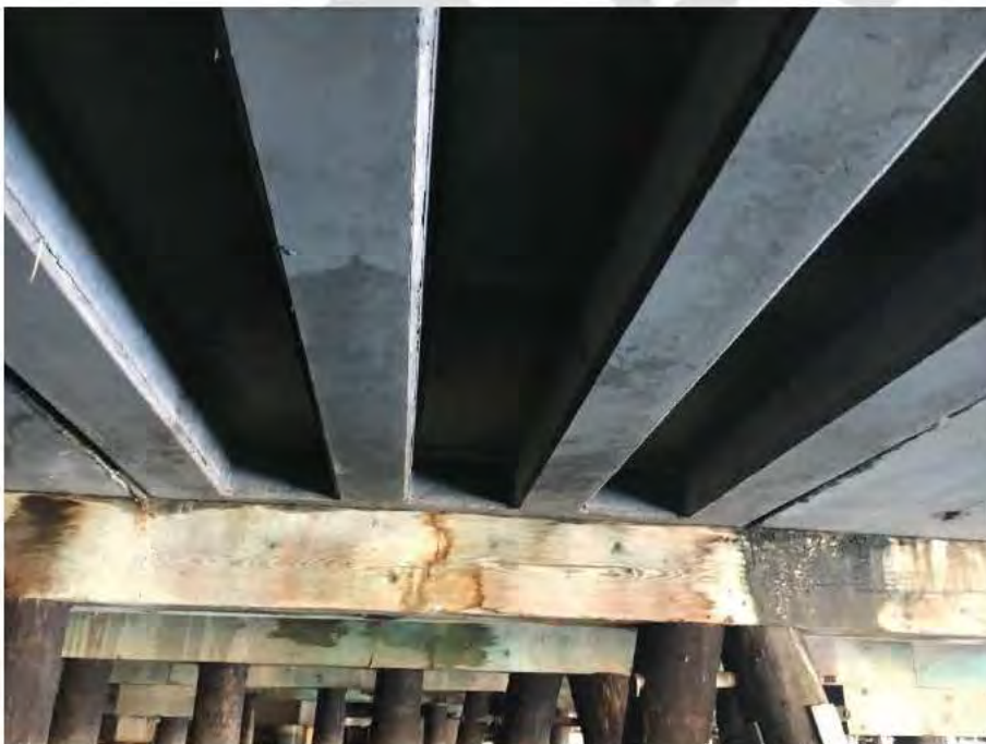
Photograph No.20: Panel No. 5 between Bent Nos 20 and 21 replaced.
