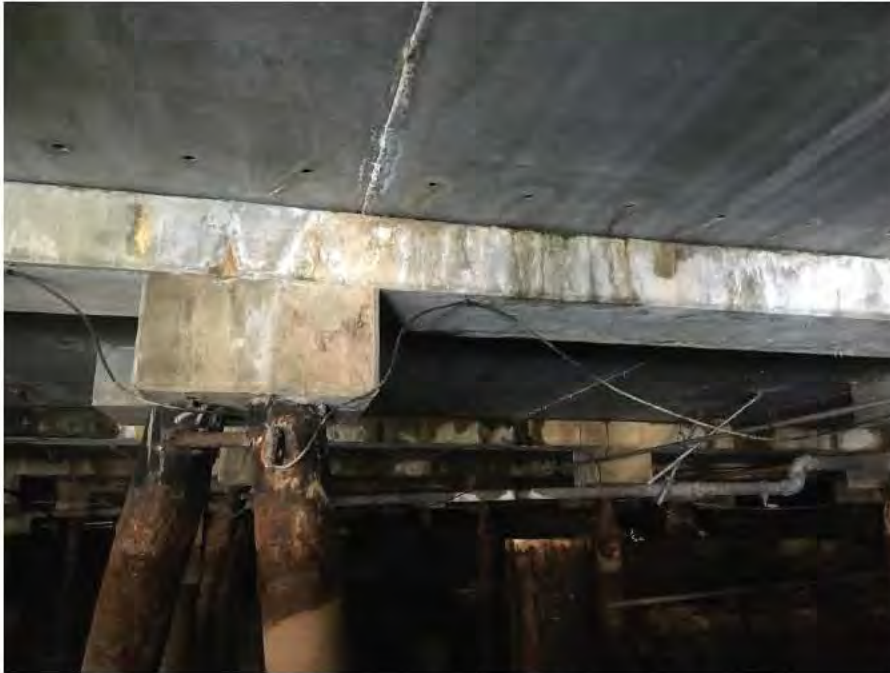
Photograph No. 3: Impressed current system installed on steel pipe piles at the City heavy deck to the southeast of Science World
