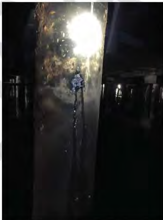
Photograph No. 2: Water ingress between pipe coating and steel pipe piles at the City heavy deck to the southeast of Science World
