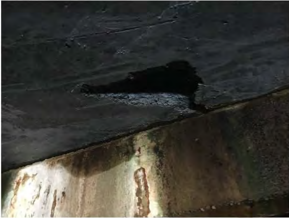
Photograph No.15: Spalling of soffit at Panel No. 11 between Bent Nos 23 and 24.
