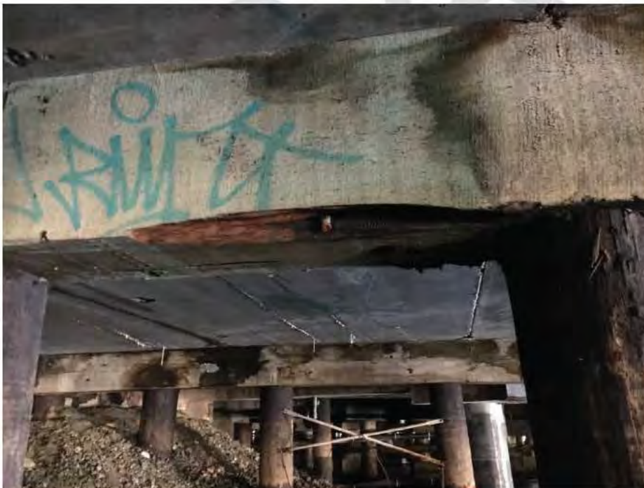
Photograph No. 8: Mechanical damage to pile cap at Bent No. 22 at location of Panel 11.
