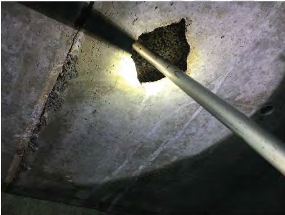
Photograph No.16: Soffit spalling at North end of Panel No. 5 between Bent Nos 22 and 23.
