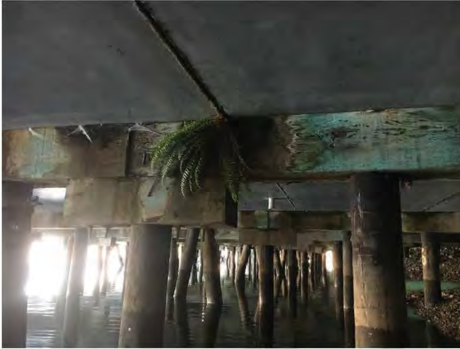
Photograph No. 9: Water ingress and vegetation growth on Pile Cap at Bent No. 18.
