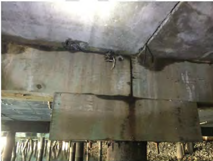
Photograph No.18: Spalled concrete at North end with exposed drift pin at Panel No. 9 between Bent Nos 21 and 22
