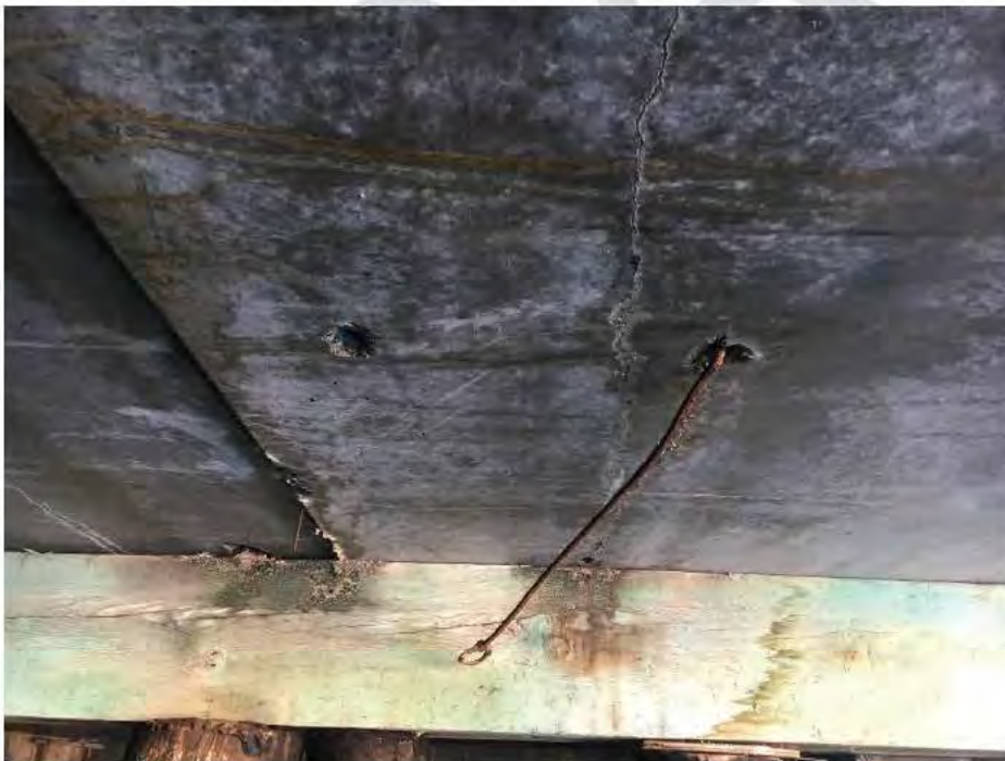
Photograph No. 10: Full length longitudinal crack and multiple spalls along the slab soffit at Panel No. 1 between Bent Nos 23 and 24.
