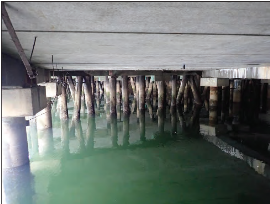
Photo 3-2 Typical View of Supporting Reinforced Concrete Substructure Located in Discrete Areas of the South Section of Substructure
