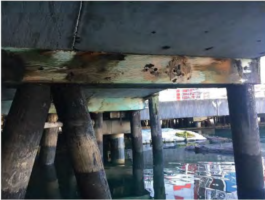
Photograph No 5: Multiple holes on side face of pile cap at Bent No. 22
