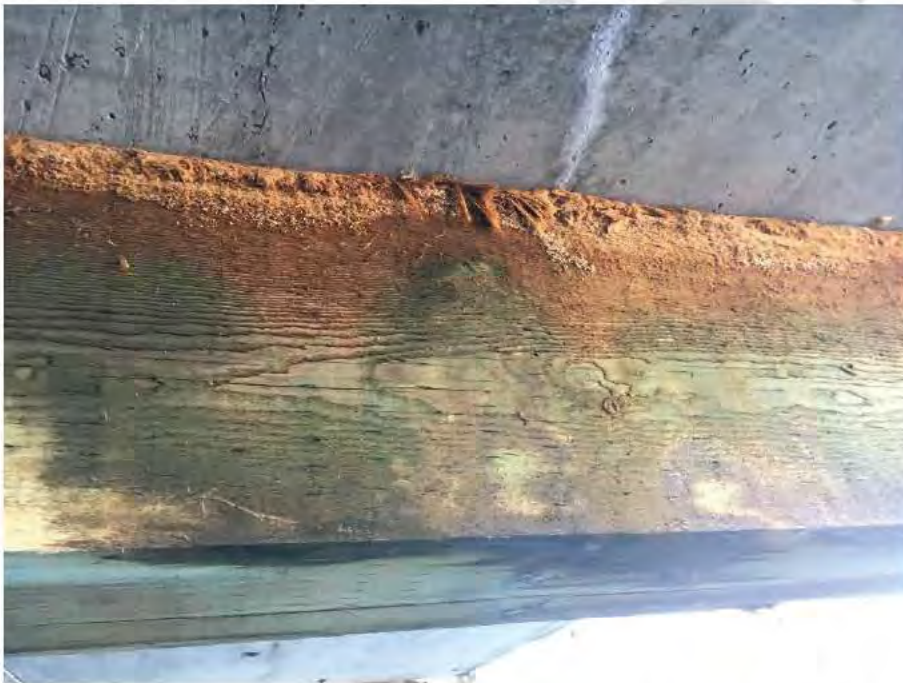
Photograph No 6: Wet internal fibres with 25 mm split at soffit of pile cap at Bent No. 22
