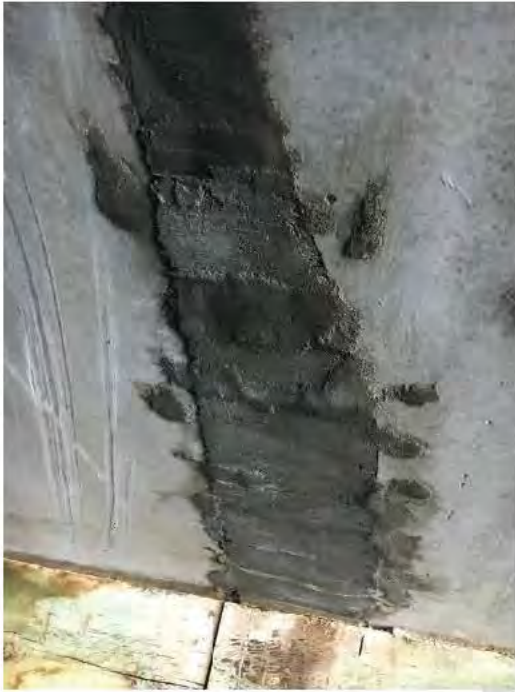
Photograph No.11: Previous grout repairs to Southeast corner of Panel No. 3 between Bent Nos 23 and 24.
