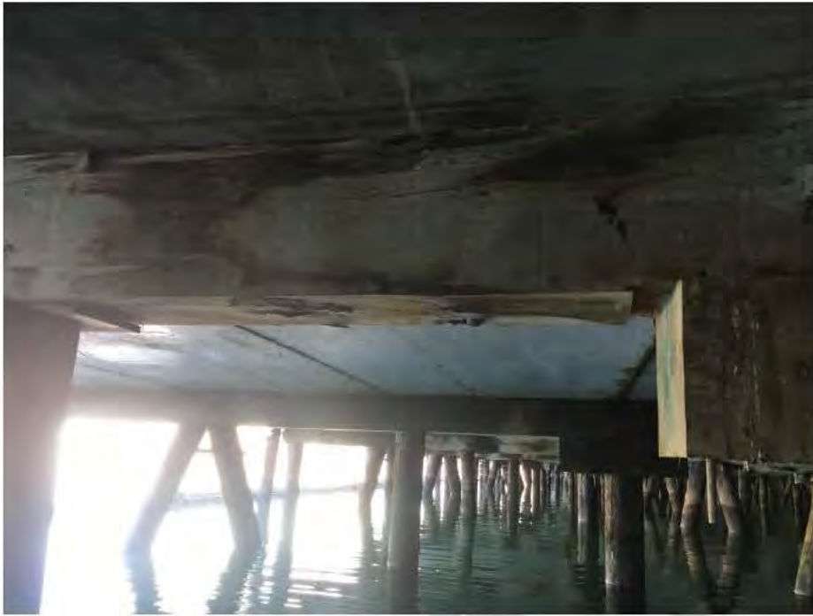
Photograph No 7: Multiple notches on pile cap at Bent No. 21
