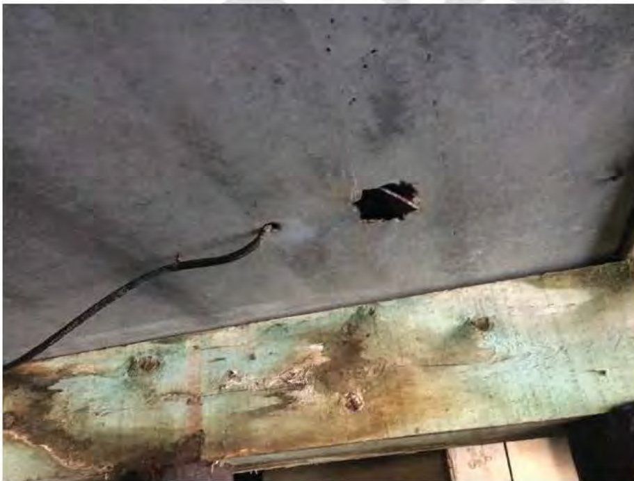
Photograph No.14: Soffit spalling at Panel No. 6 between Bent Nos 23 and 24.
