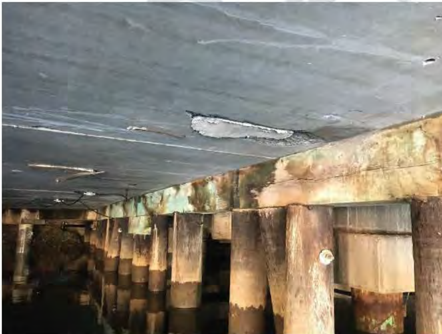
Photograph No.12: Previously installed repair at Southeast corner of Panel No. 4 between Bent Nos 23 and 24 failing.
