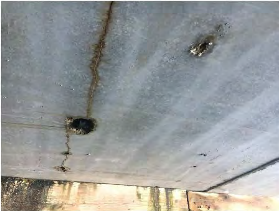
Photograph No.19: Spalling of deck soffit and cracking with efflorescence at Panel No. 4 between Bent Nos 20 and 21.
