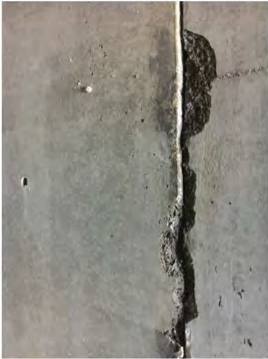
Photograph No.17: Spalling of deck soffit at interface of Panel Nos. 5 and 6 between Bent Nos 21 and 22.
