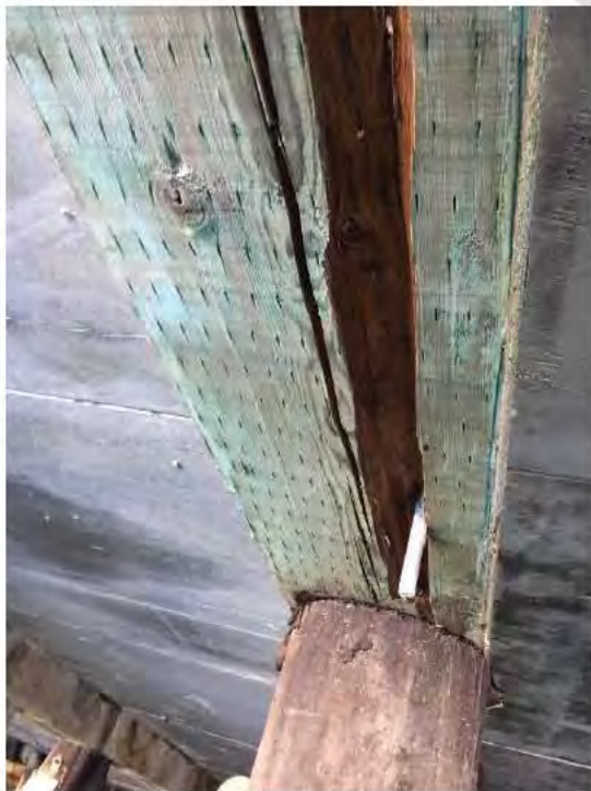
Photograph No. 4: Mechanical damage to pile cap at Bent No. 22.
