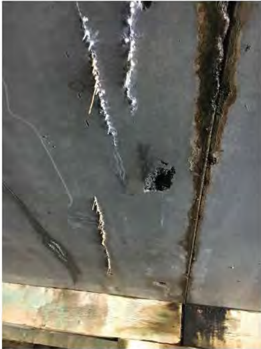
Photograph No.21: Spalling of deck soffit and cracking with efflorescence at Panel No. 7 between Bent Nos 20 and 21.
