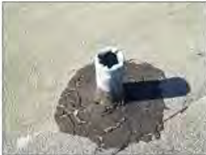
An example of lead flashing around exhaust pipes on the roof.
