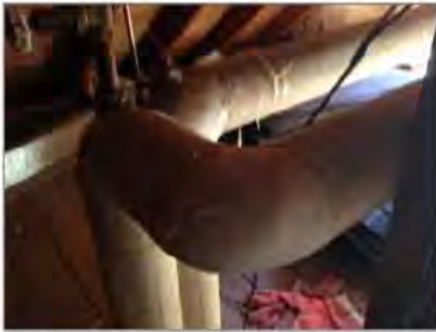
Unlabelled asbestos-containing pipe elbows.
