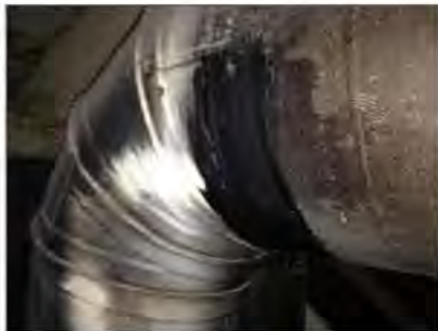
Asbestos-containing black duct mastic.
