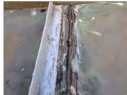
Asbestos-containing silver duct mastic.
