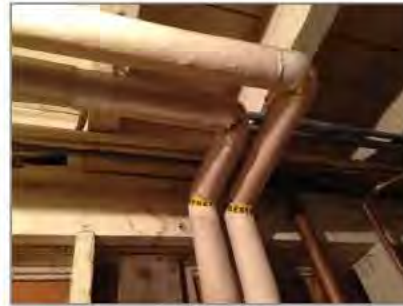
Labelled asbestos-containing pipe elbows.
