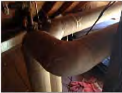
Unlabelled asbestos-containing pipe elbows.
