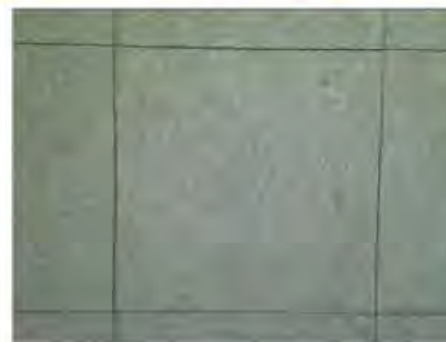
Non asbestos floor tiles concealing asbestos-containing mastic.
