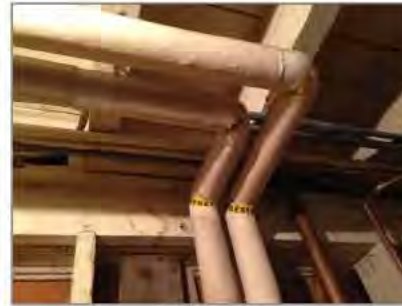
Labelled asbestos-containing pipe elbows.
