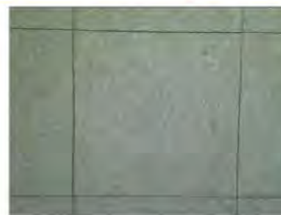
Non asbestos floor tiles concealing asbestos-containing mastic.
