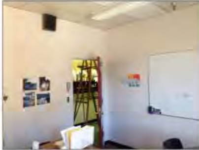
Drywall walls with asbestos-containing joint compound.
