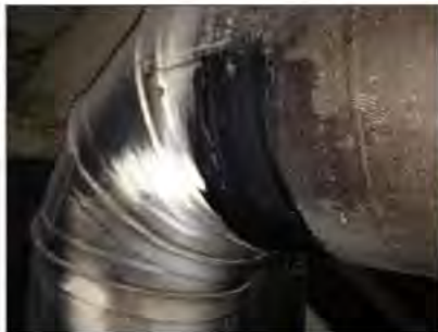
Asbestos-containing black duct mastic.
