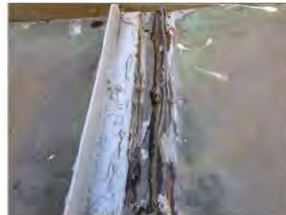
Asbestos-containing silver duct mastic.
