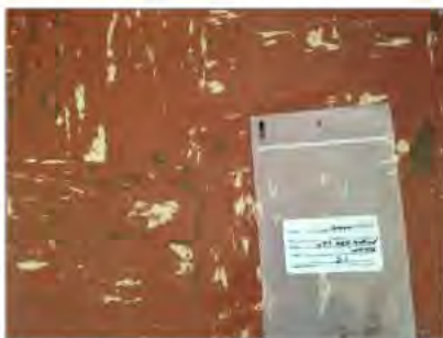
Asbestos-containing vinyl floor tiles.
