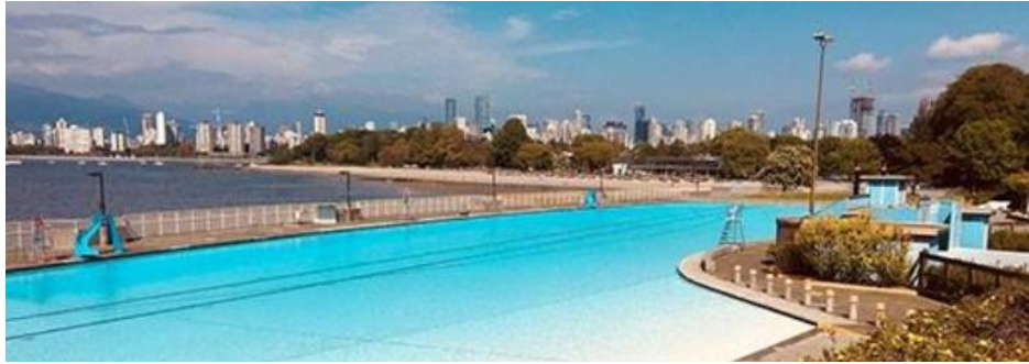
Figure 1 – Image of Existing Kitsilano Outdoor Pool
