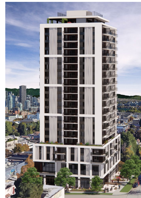
2079-2085 W 5th Ave – 200 social housing units with ground floor commercial space & offices.
