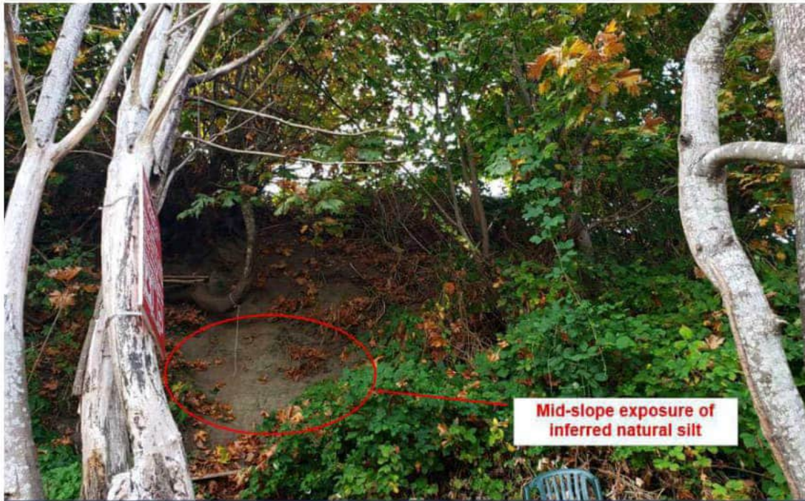
Photograph 6: Existing Condition of South Slope (looking south and upslope from beach)
