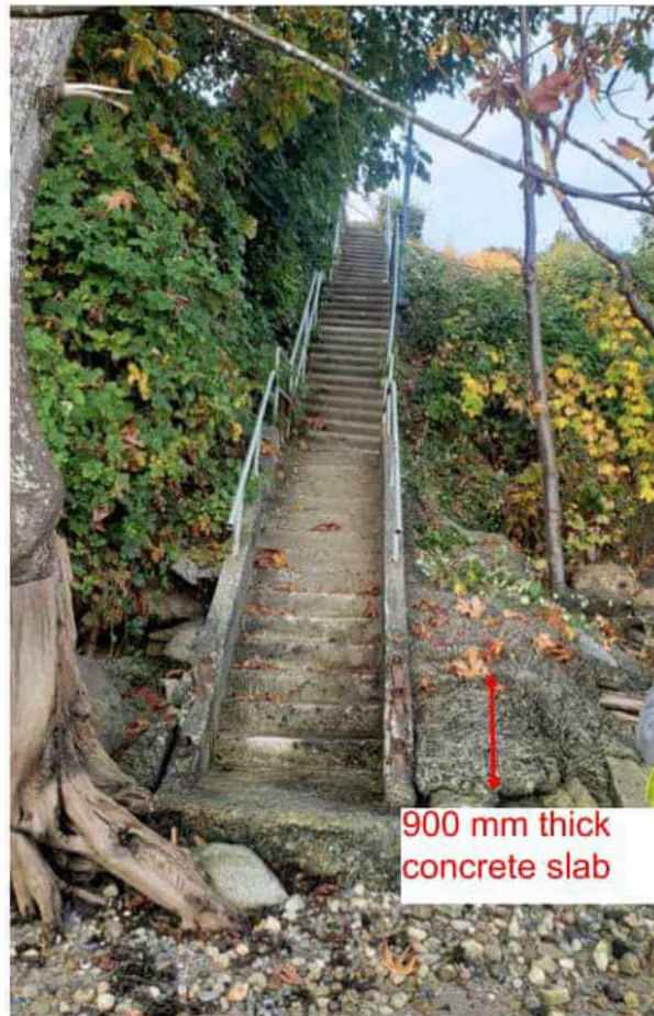
Photograph 8: Existing condition of beach access staircase, looking up from bottom
