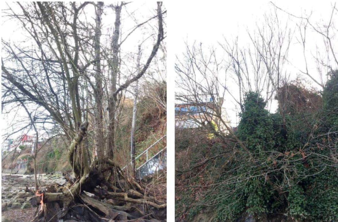
Figure 4. Trees at the toe of slope (left - #15); and infested with English ivy into the crown (right - Tree #4)
