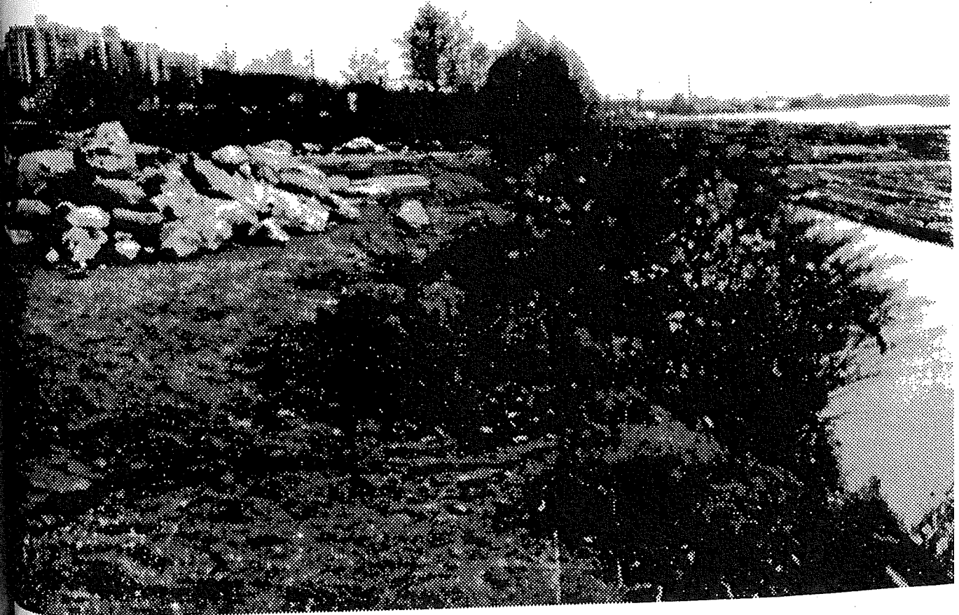
bank east of North Arm Transportation (looking east)
